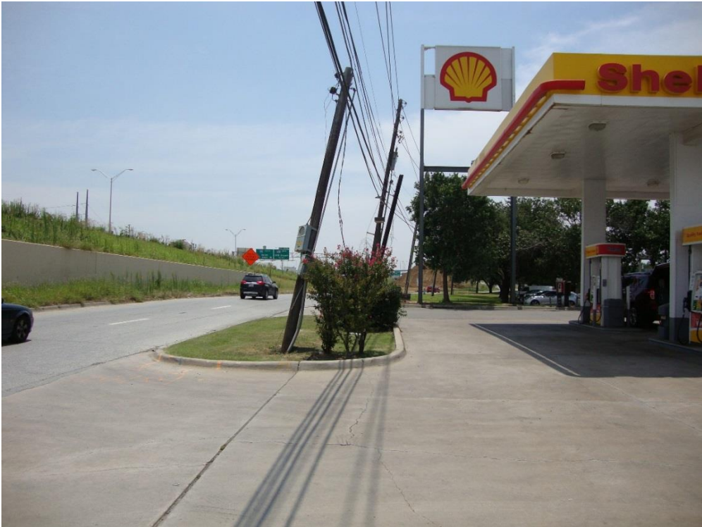
View along Stemmons Freeway, Southbound frontage road
