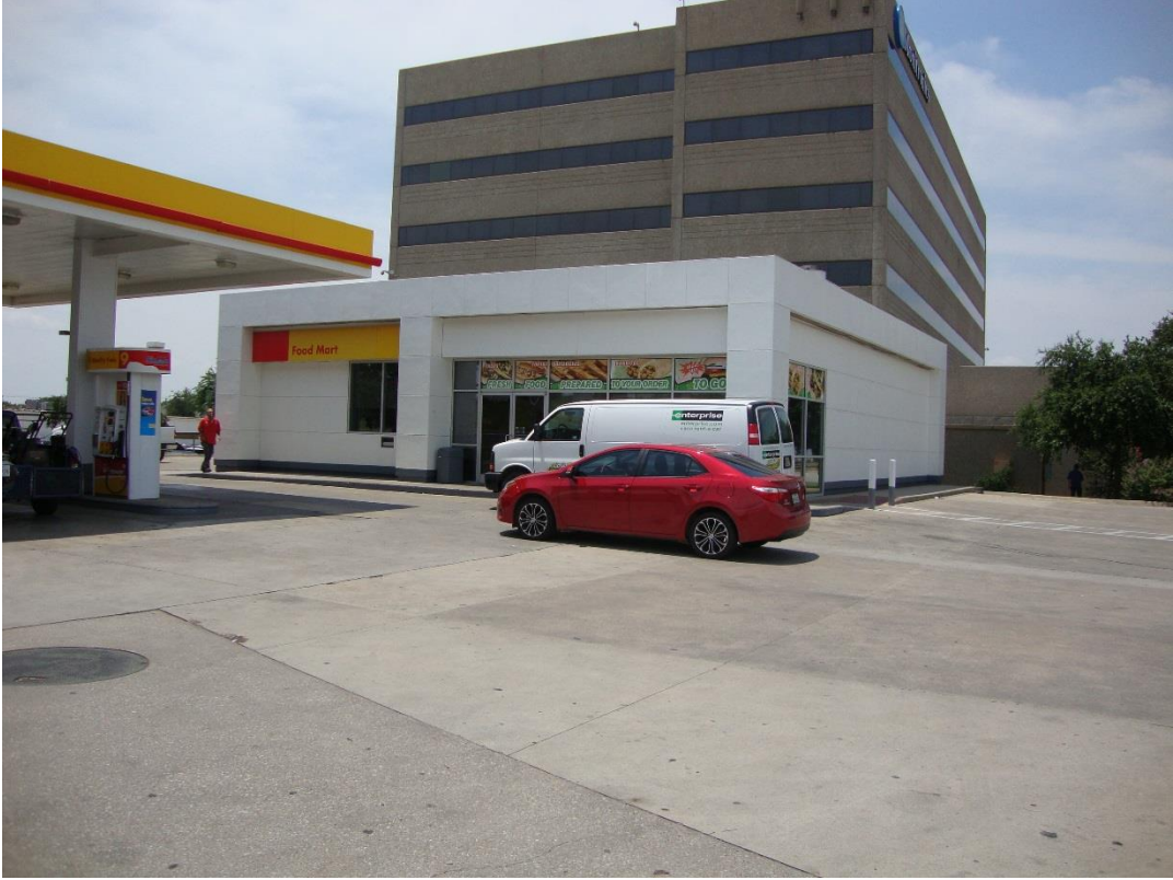
View from Stemmons Freeway, facing Southwest
