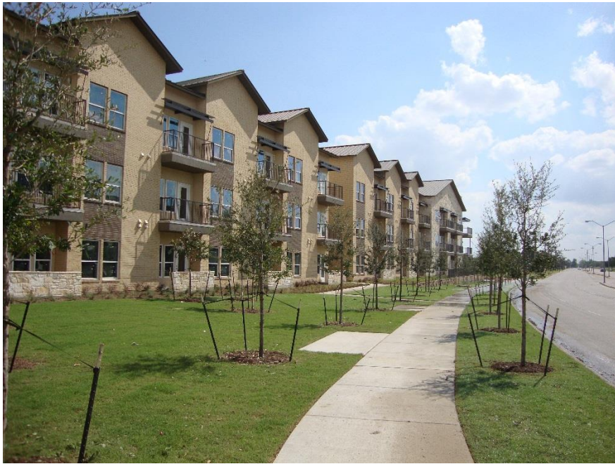
Facing south along Luna Road at the constructed Phase One project
