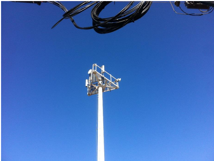
Existing bracket and cellular equipment on tower
