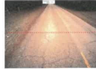
Crack-Block – Severe
