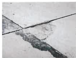
Corner Spalling
