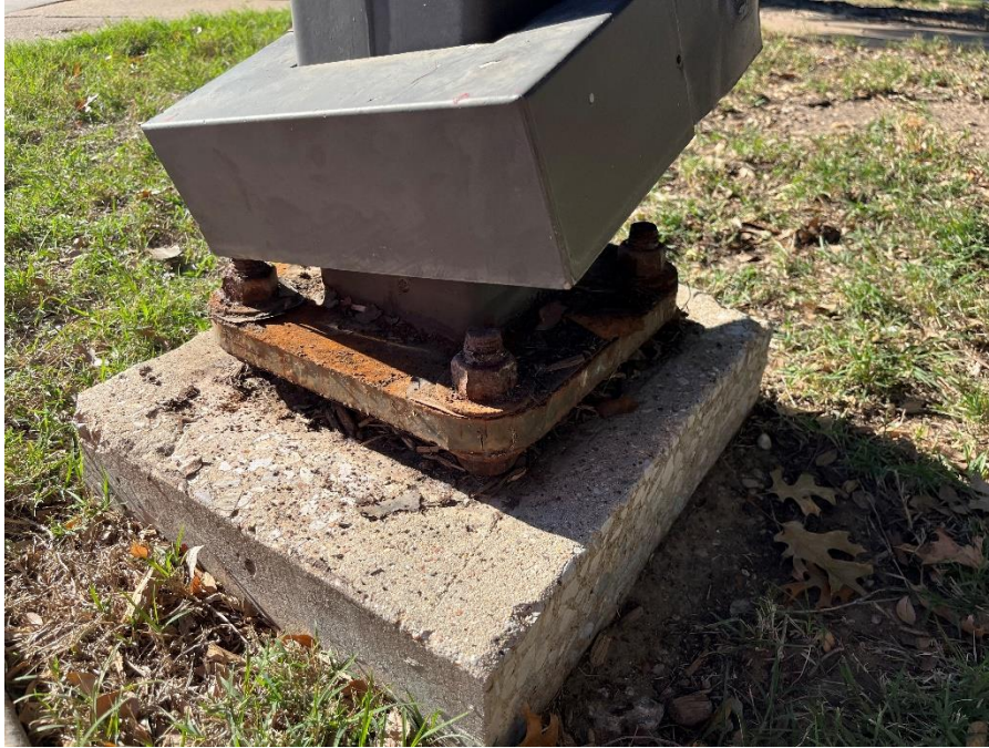
Figure 21. Typical 31-foot light pole base at Morningstar Park (MOP 2).
