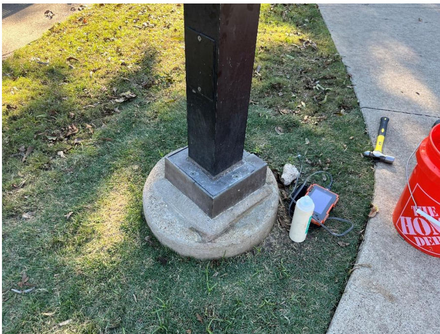
Figure 3. Typical base of a 16-foot aluminum pole at Gussie Field Watterworth Park (GP 29).
