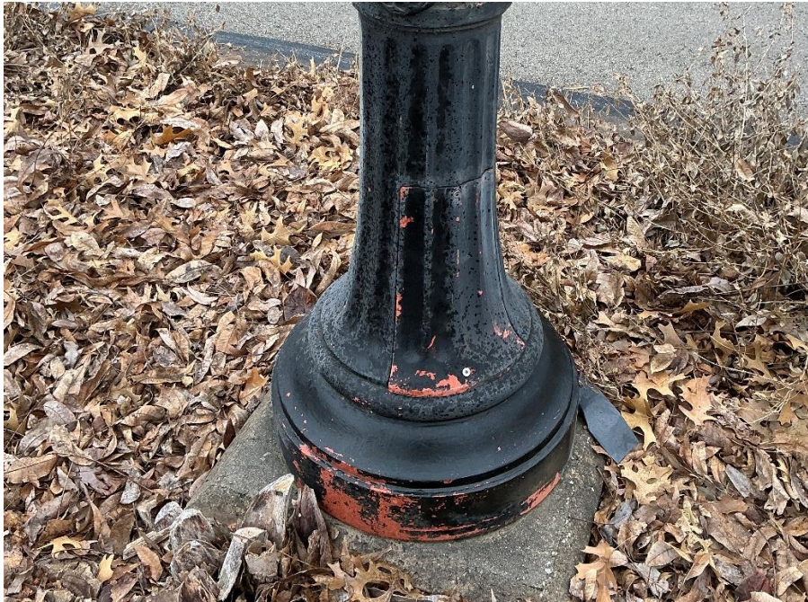
Figure 6. Typical base of a 15-foot aluminum pole at Gussie Field Watterworth Park (GP 32).
