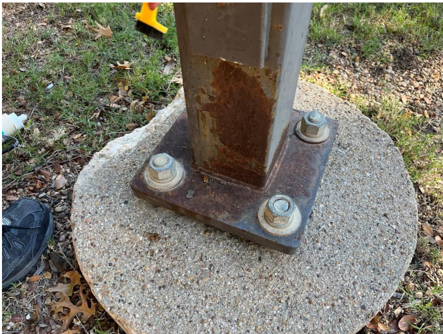
Figure 14. Severe Corrosion at the base of pole SP 6 at Squire Park.
