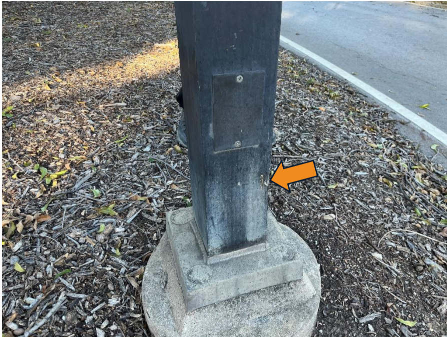
Figure 2. Typical base of a 29-foot aluminum pole at Gussie Field Watterworth Park (GP 1). The orange arrow indicates dent in pole shaft.
