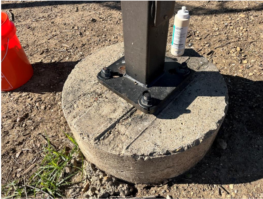
Figure 17. Typical 24-foot light pole base at Jaycee Park (JP 3).
