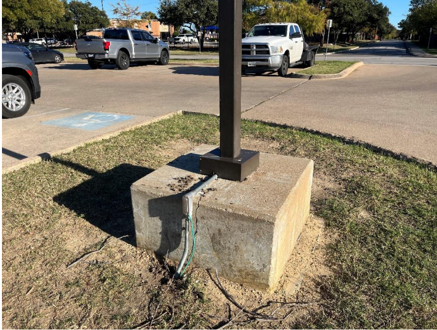
Figure 11. Typical 14-foot light pole base at Farmers Branch Park (FB 1).
