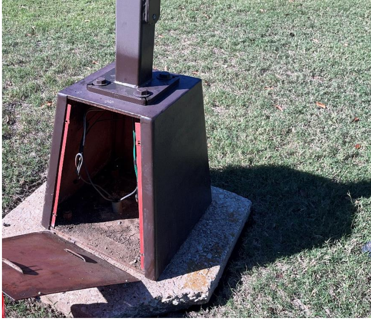
Figure 25. Typical 25-foot light pole base at Dutch Village Park (DV 1).
