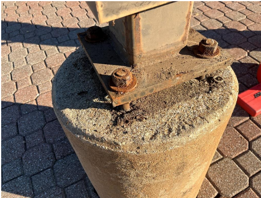
Figure 16. Typical 30-foot light pole base at Jaycee Park (JP 5).
