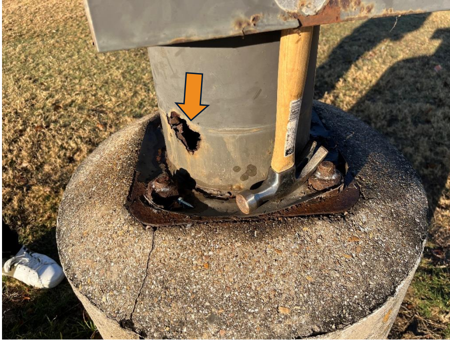
Figure 9. Through-thickness corrosion (orange arrow) at base of Pole OP 3 at Oran Good Park.
