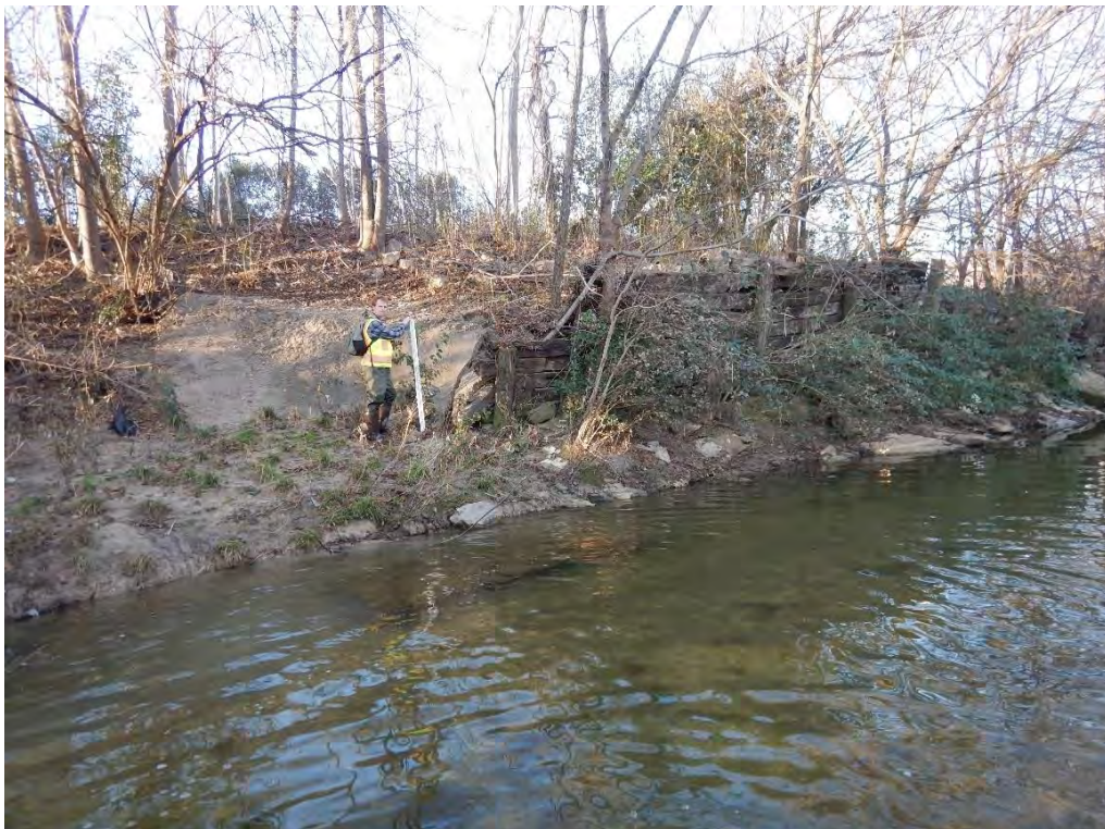
Photo 20. A degrading timber and concrete wall on the left bank may be protecting a Valley View Lane or a sewer line (photo taken looking at the left bank).
