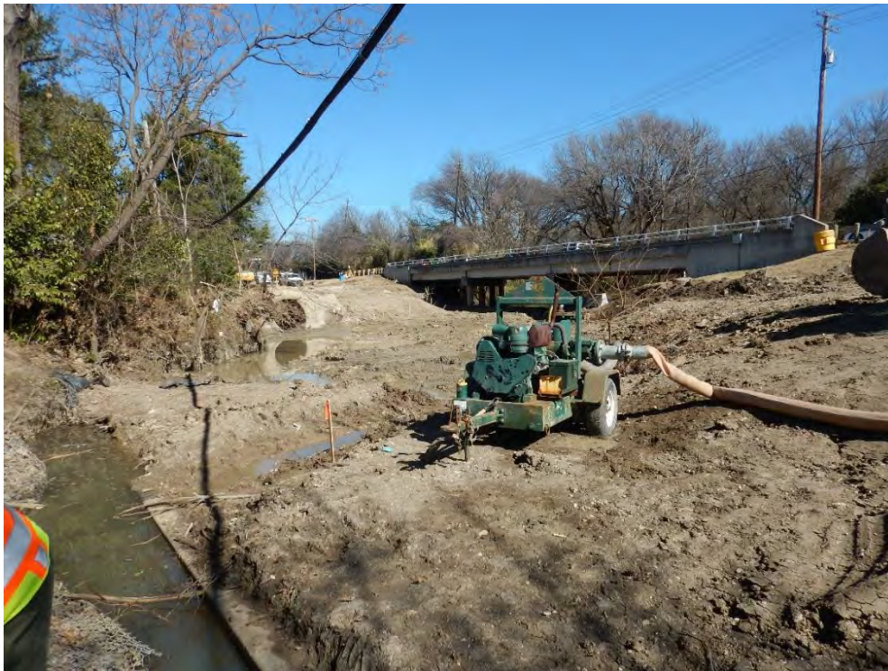
Photo 8. Construction access and a coffer dam were built for the new bridge. The observed conditions during the site visit may not be representative of normal conditions. FNI recommends monitoring upstream conditions after coffer dam removal (photo taken looking upstream).
