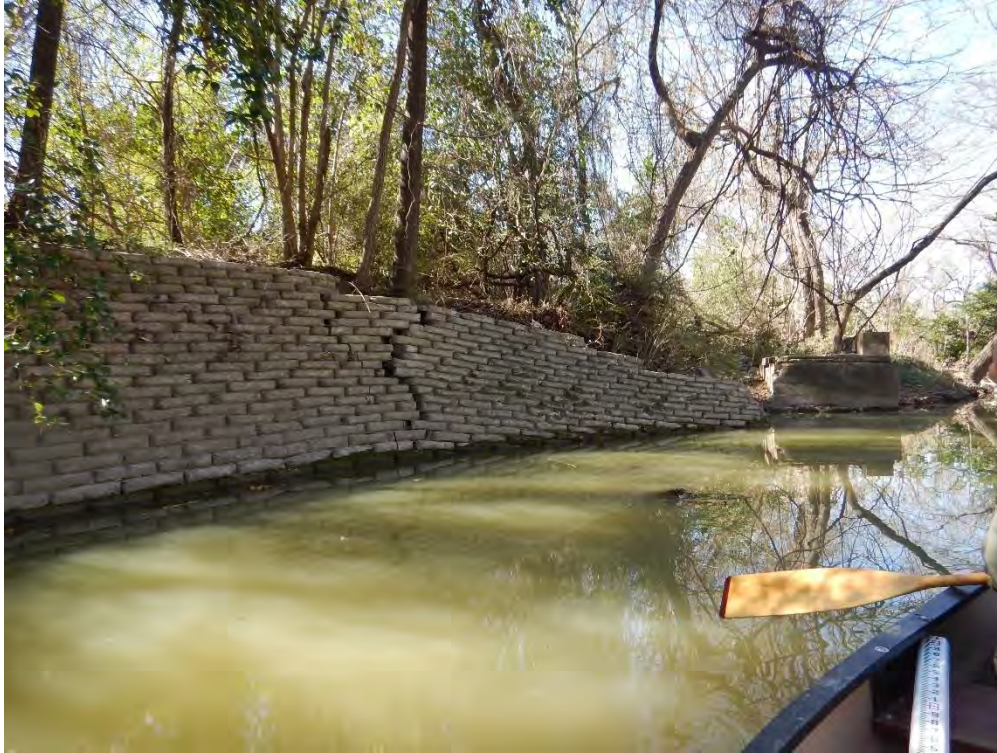
Photo 9. A bag wall on the left bank is cracked and leaning. No undercutting was observed (photo taken looking at the left bank).
