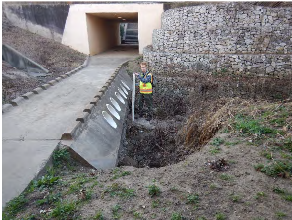
Photo 18. A deep gully is undercutting a trail crossing near Valley View Lane in Mustang Trails Park. The gully meets Farmers Branch Creek at the right edge of the photo, which continues flowing to the right (photo taken looking at the left bank). Valley View Lane runs above the tunnel shown in the photo as well as over a bridge just behind the cameraman.
