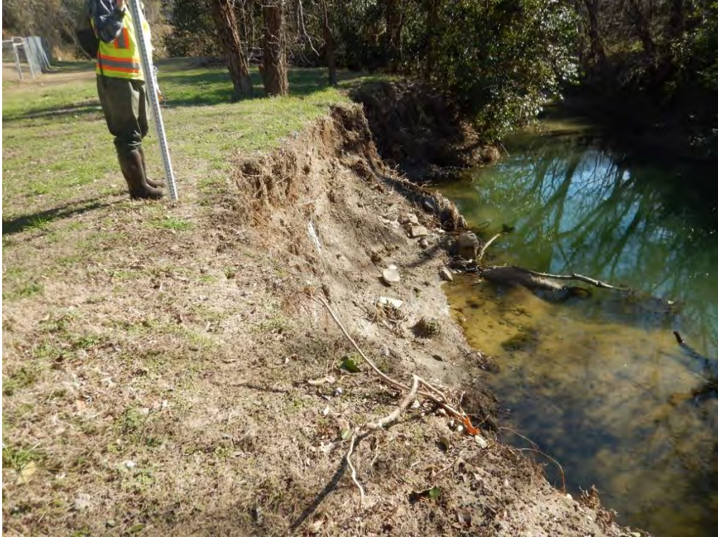
Photo 35. This south-facing, bare right bank (10 feet tall) has high erosion potential. Tension cracks were observed within 6 inches of the top of the bank (photo taken looking upstream along the right bank).
