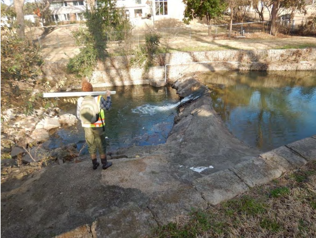
Photo 23. A degrading concrete drop with a deep pool on the downstream side (photo taken looking at the right bank). It is recommended that an engineer assess the condition of this structure.
