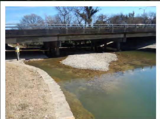
Sediment deposition extends into Mallon Park pond
