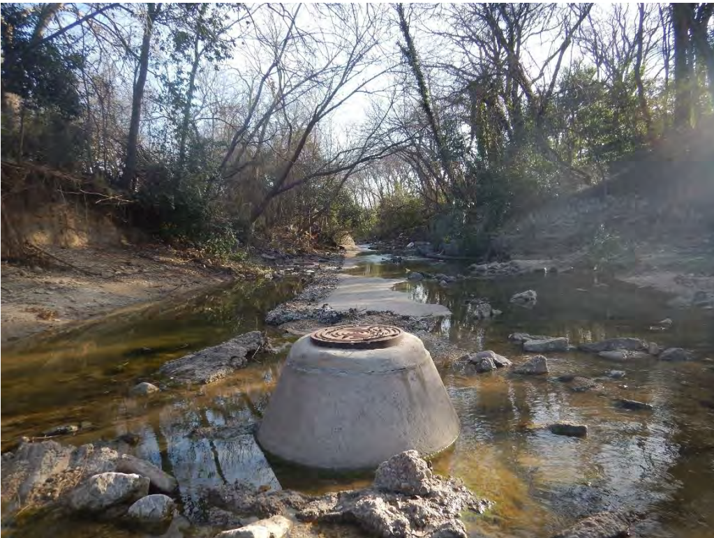
Photo 24. Manhole in center of channel at a junction of three pipelines (photo taken looking upstream).
