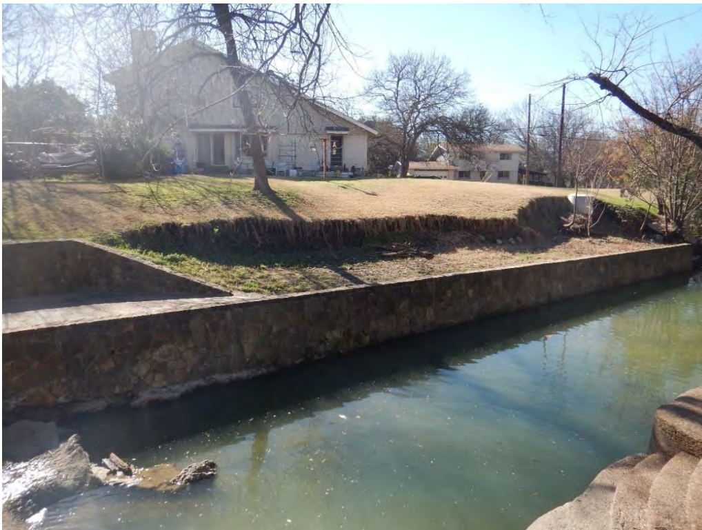
Photo 38. A manhole riser is exposed on a scoured left bank above a retaining wall (photo taken looking at the left bank). No undercutting was observed along the retaining wall.
