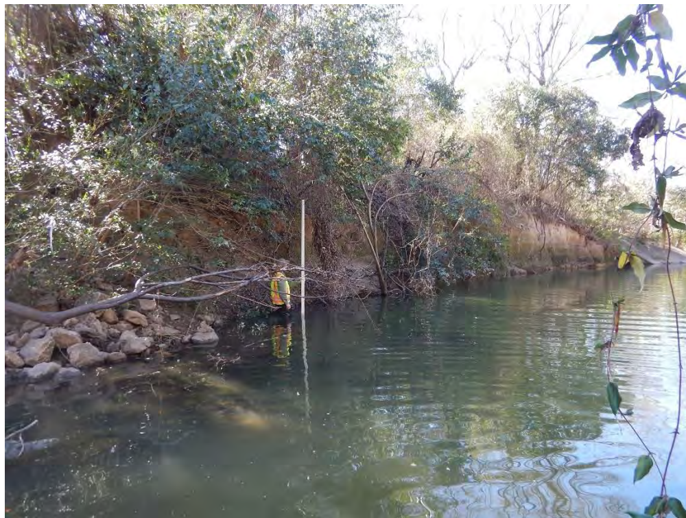
Photo 12. Erosion of the left bank is encroaching on Valley View Lane, located at the top of the bank (photo taken looking downstream along the left bank).
