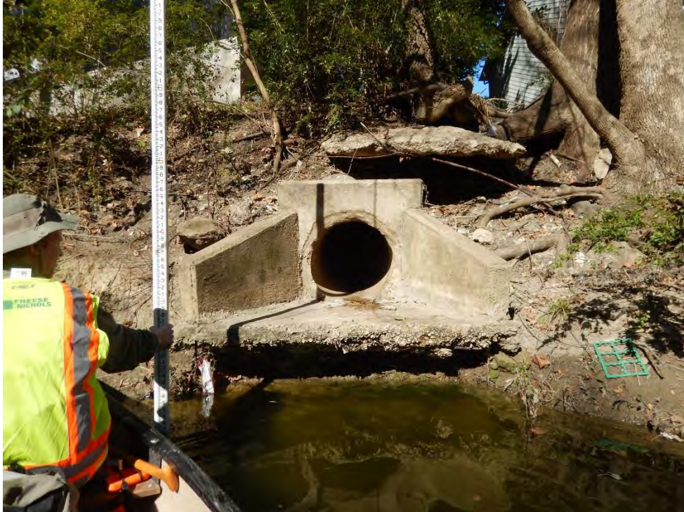
Photo 7. A stormwater headwall on the right bank has been undercut by 2 feet. The pipe is 18 inches in diameter, and there is a 1-foot deep pool at the base of the outfall (photo taken looking at the right bank).
