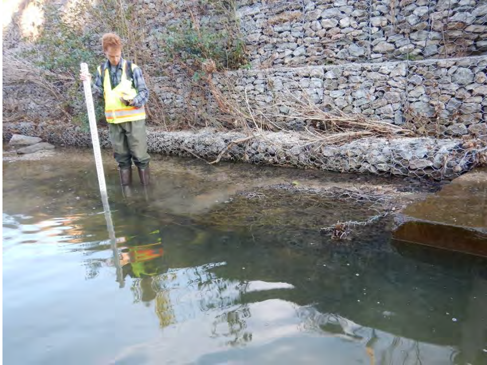
Photo 19. Minor damage to gabion mattress downstream of outfall (photo taken looking at the right bank). Maintenance is recommended.
