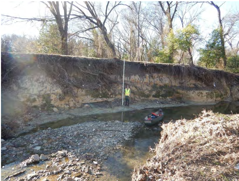
Photo 2. Bare, near-vertical, 15-foot tall left banks near Brookhaven College have high erosion potential (photo taken looking at the left bank).
