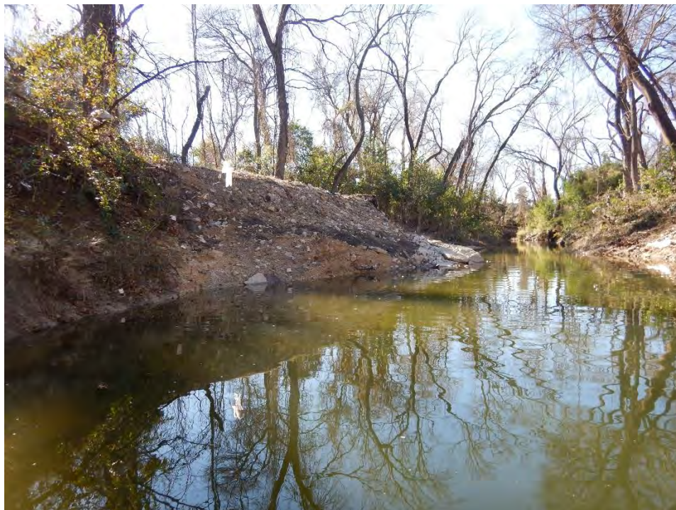
Photo 4. Fill placed on the left bank at an outfall. This is acting as a flow constriction (photo taken looking downstream).
