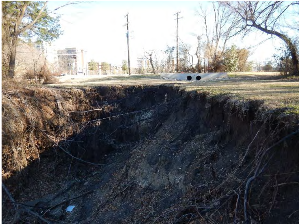
Photo 1. Eroding left bank near the upstream city limits. A headcutting gully has formed by a stormwater outfall 50 feet from the top of bank (photo taken looking at the left bank).
