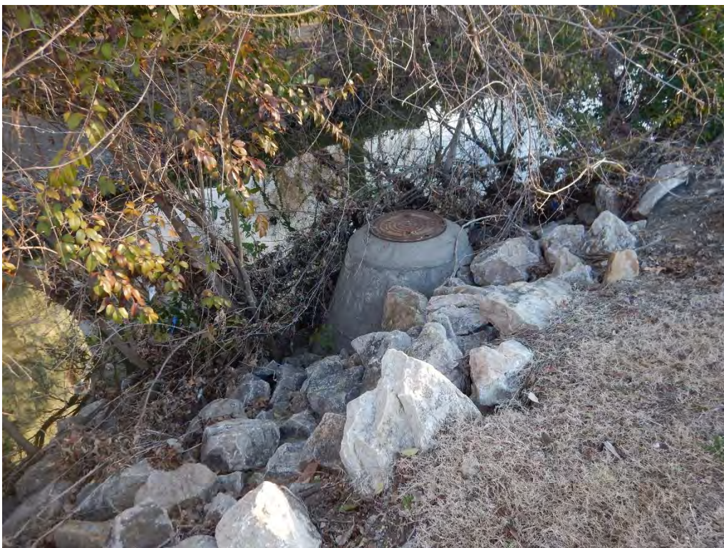
Photo 16. A manhole next to the creek protected with riprap (photo taken looking into the channel from the top of the right bank). This is no immediate threat, but it should be monitored.
