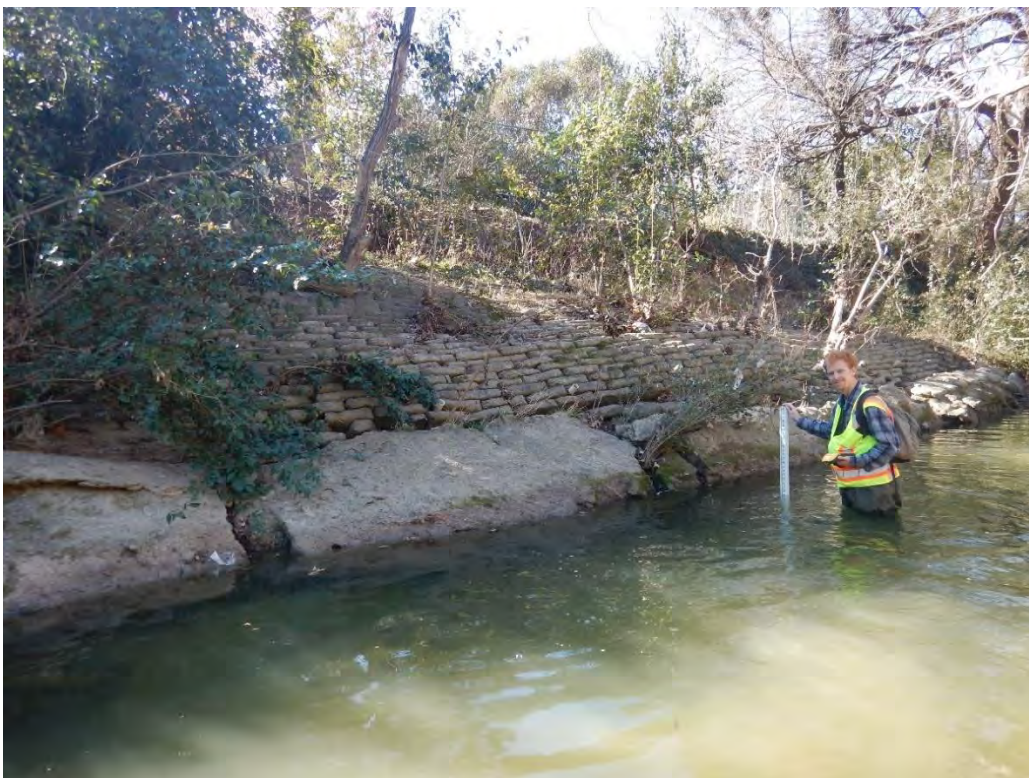
Photo 36. An old slump with a collapsed bag wall on the left bank. A chainlink fence at the top of the bank was damaged (photo taken looking at the left bank).
