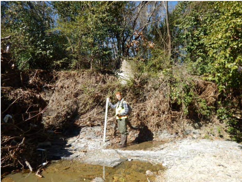
Photo 40. A manhole riser is less than 5 feet from being exposed on the right bank (photo taken looking at the right bank). It is recommended that a utility engineer check the alignment and consider bank protection.
