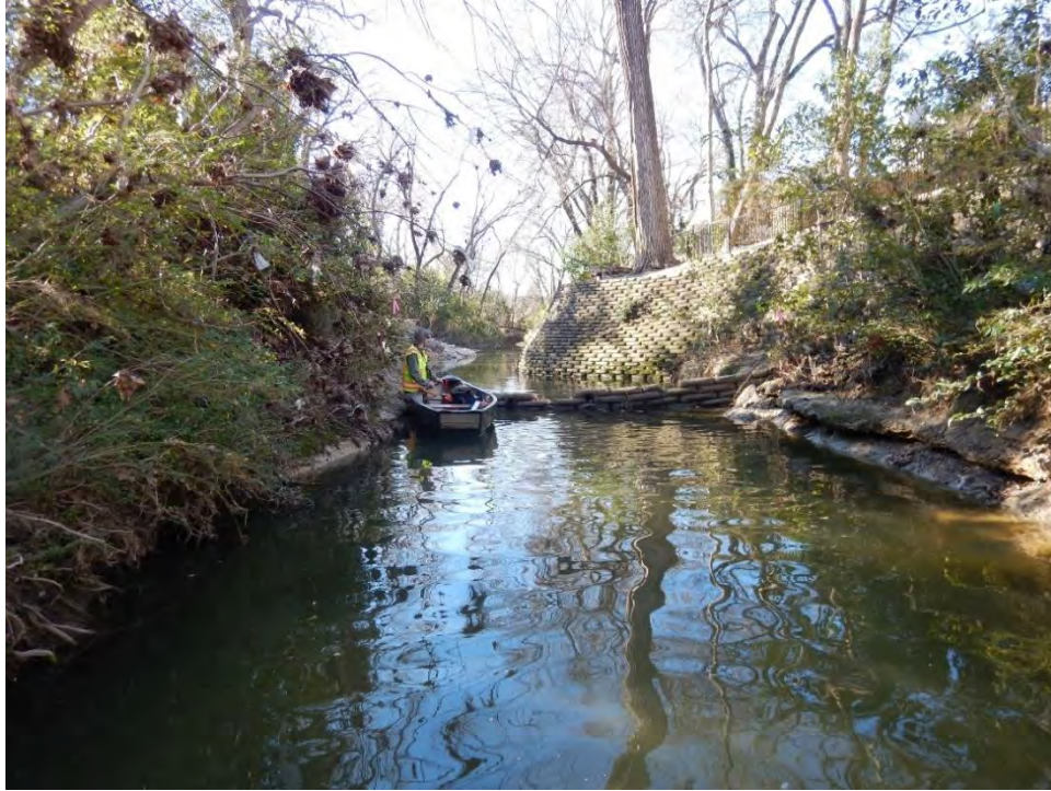
Photo 3. A degraded bag wall structure in the channel. No undercutting was observed, but there is a deep pool (3 feet) on the downstream side (photo taken looking downstream).
