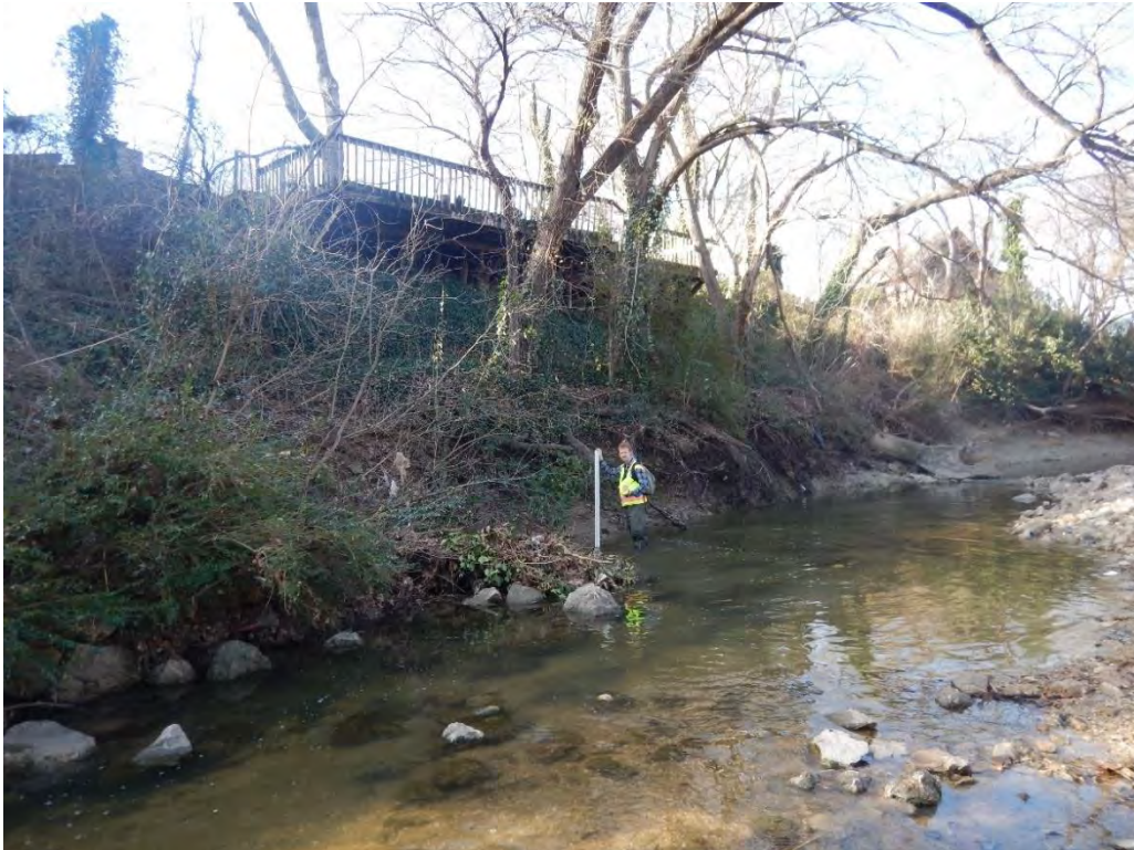
Photo 27. A deck at the top of a steep section of the left bank is overhanging the creek (photo taken looking downstream along the left bank).
