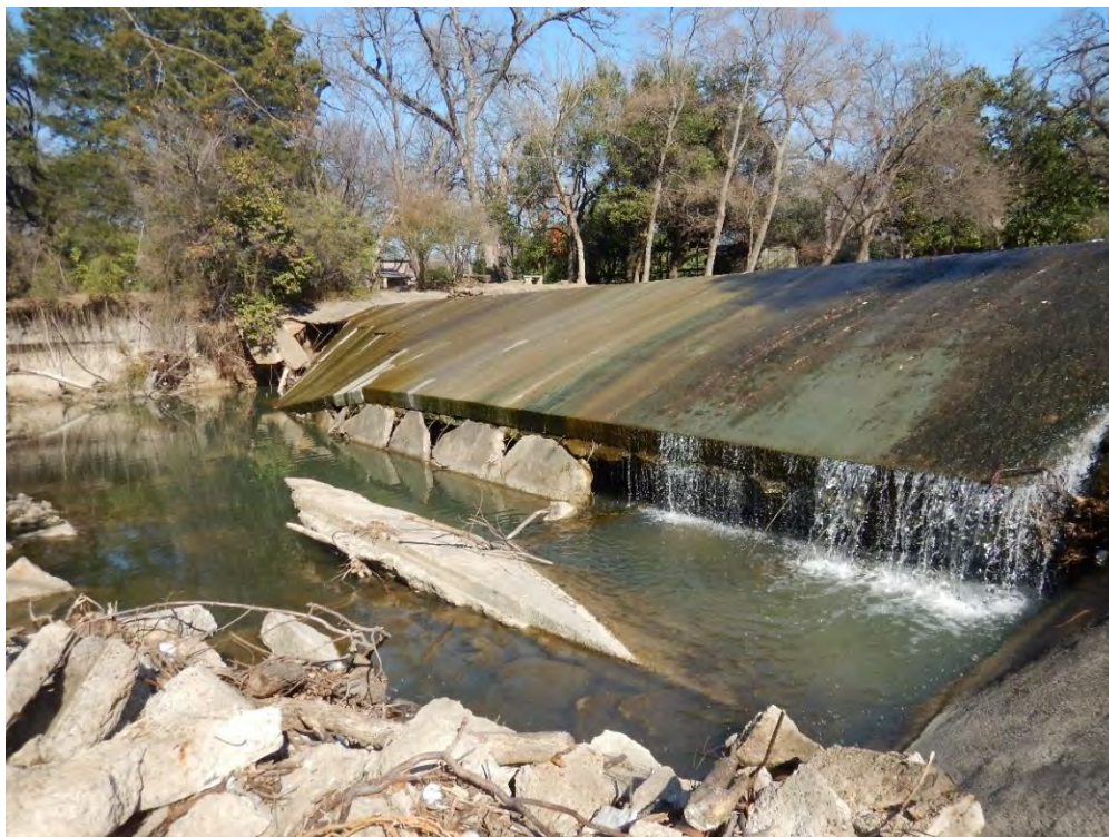
Photo 48. This dam is cracked and collapsing (photo taken looking in the upstream direction). A homeowner repaired it in April 2016. There is also an exposed pipeline underneath the dam. It is recommended that an engineer assess the condition of the dam.
