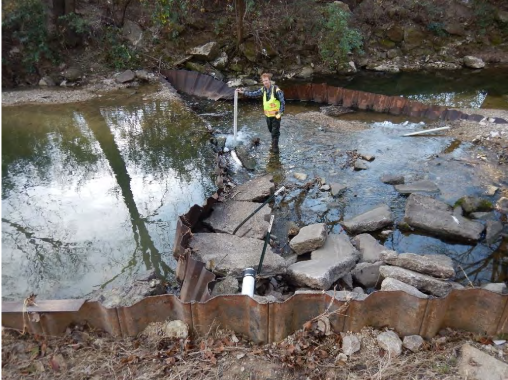
Photo 21. A damaged sheetpile check dam with a broken, PVC-capped pipe on the downstream edge (photo taken from the right bank; the creek flows to the right).
