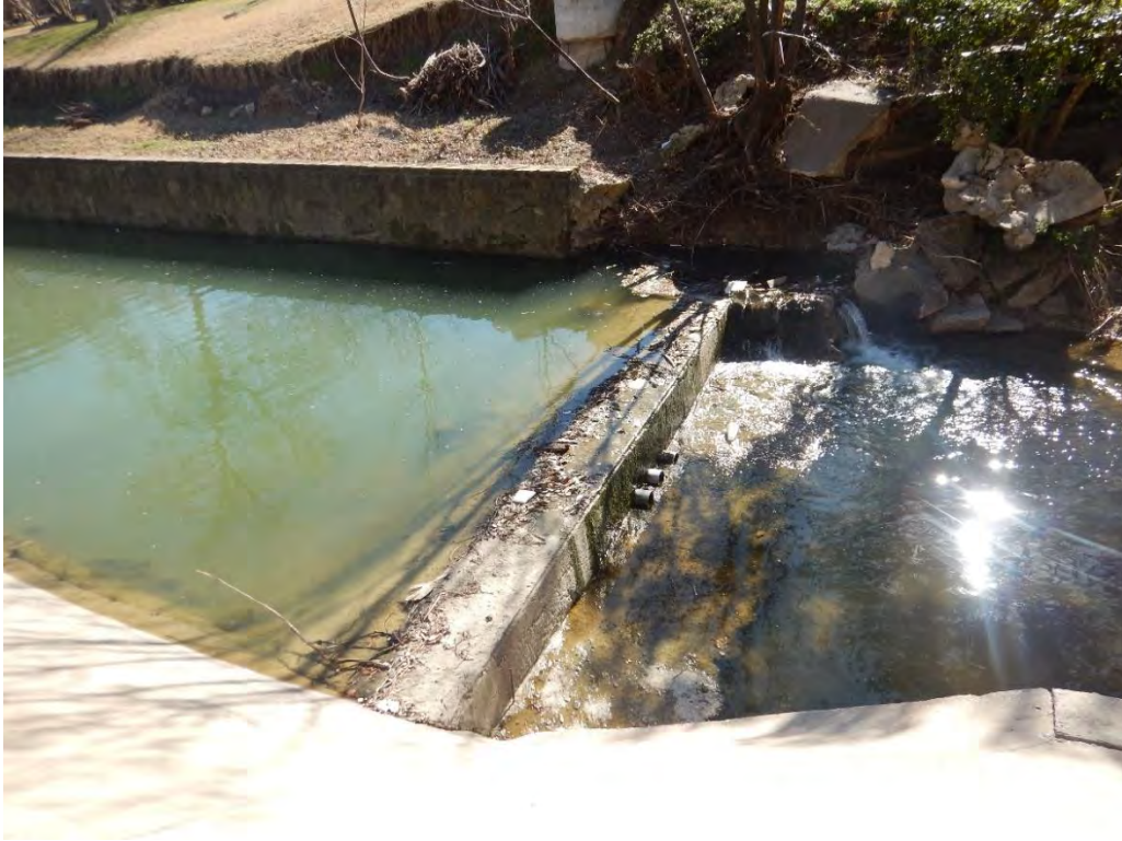
Photo 39. Water is beginning to flow around this grade control structure where the concrete protection ends, eroding the left bank (photo taken looking at the left bank).
