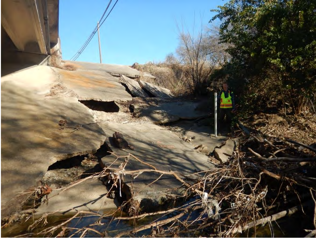
Photo 31. Concrete apron collapsed on the right bank upstream of Webb Chapel Road due to scour (photo taken looking at the right bank).
