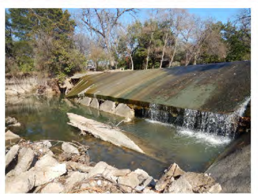
Dam collapsing and breached on left side; exposed pipe under dam; engineer should assess condition
