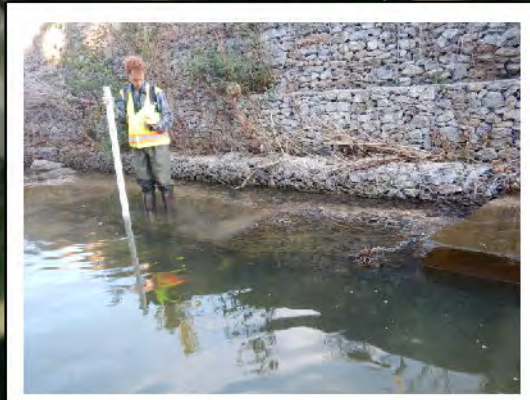
Minor damage to gabion mattress downstream of outfall
