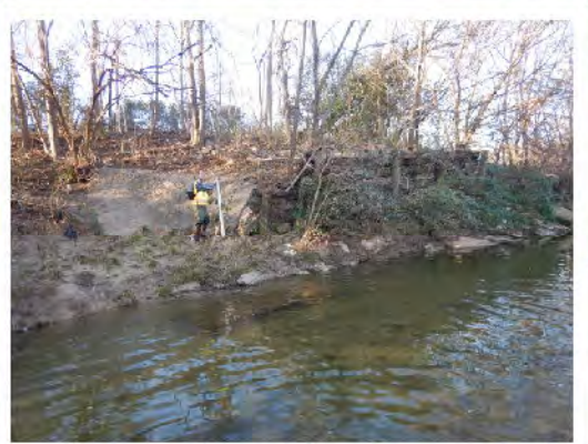
Old timber wall on left bank is rotting and leaning
