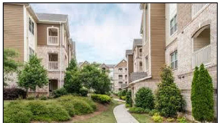
Internal sidewalks provide connections between parking, amenities, and buildings.
