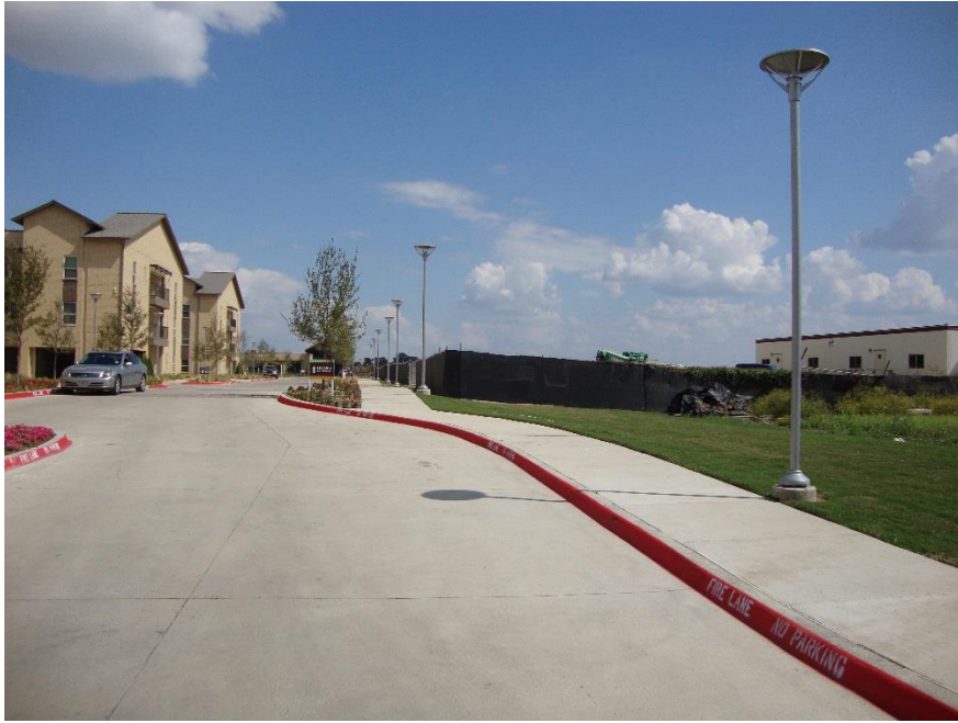
Facing east at the dividing street between Phase One and Two
