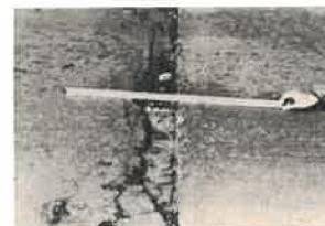
Joint Spalling
