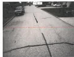
Crack-Seal - Example 2
