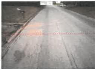
Crack-Block – Minor
