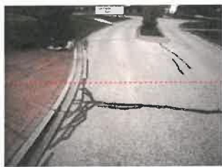
Crack-Seal - Example 1
