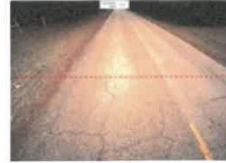
Crack-Block – Severe
