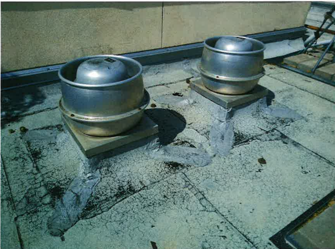
Overview of exhaust base flashings.
