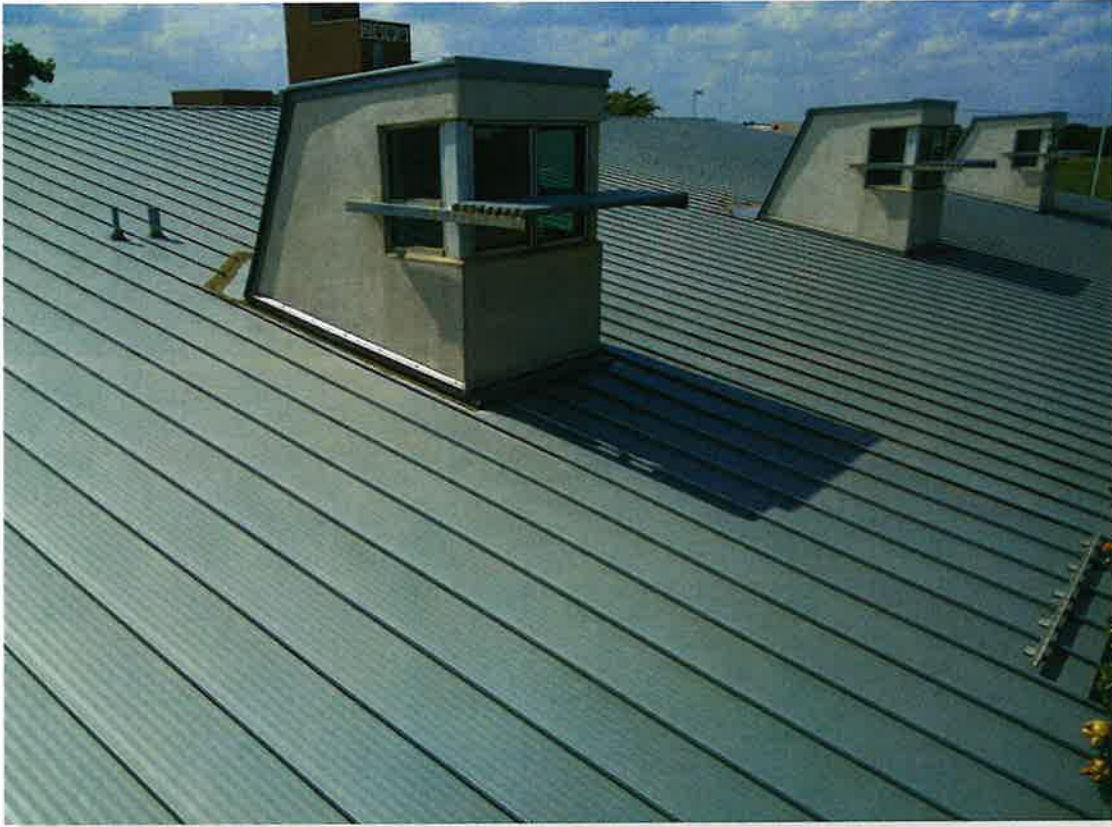
Overview of metal roof section.
