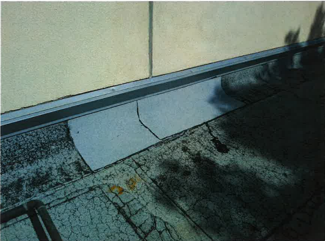
Previous wall flashing repair.
