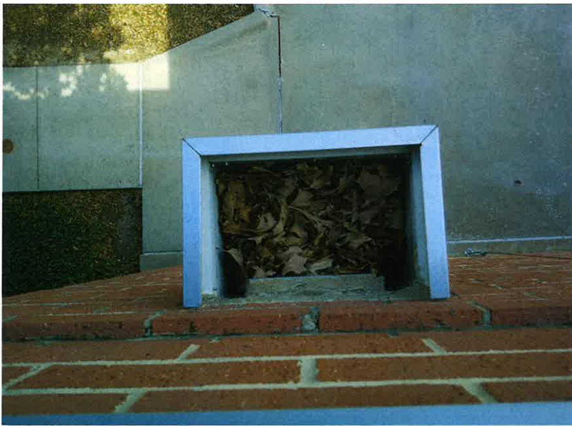
Leaf debris in conductor head.
