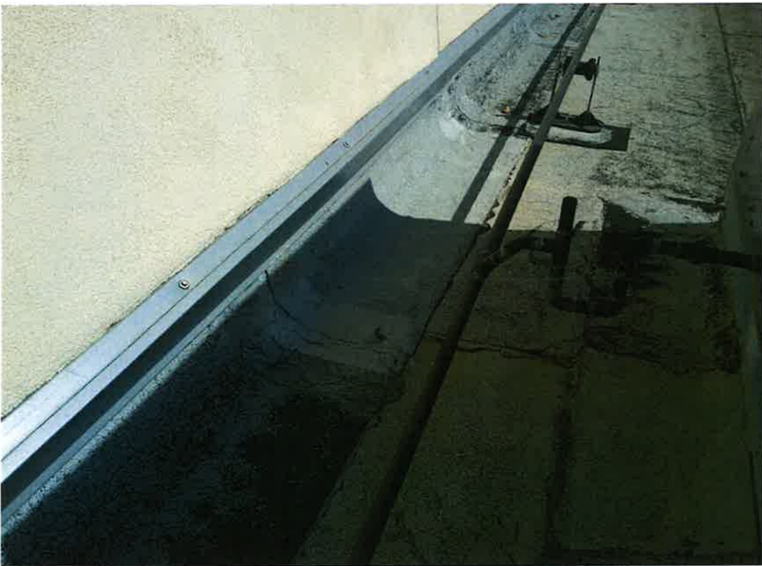
Previous wall flashing repair.
