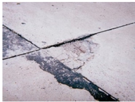
Corner Spalling
