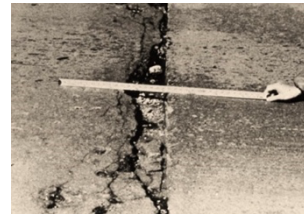
Joint Spalling
