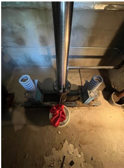
15. City Hall – Car 2 – View of pit. (spring buffers, hydraulic jack, and overflow bucket).
