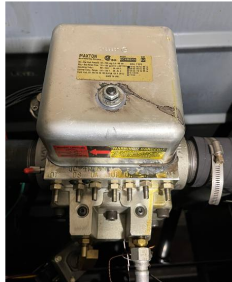
34. Menske Library – Maxton UC 4 hydraulic valve. (Controls the direction of the hydraulic jack).
