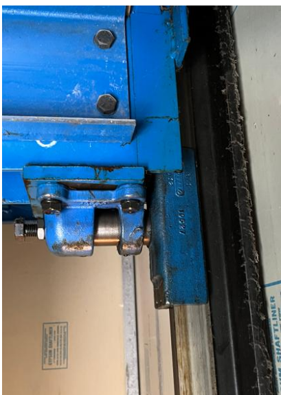
27. City Hall – Car 2 – Slide guides on car. (bottom)
