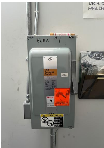
3. City Hall – Car 1 – High Voltage Disconnect for elevator.
