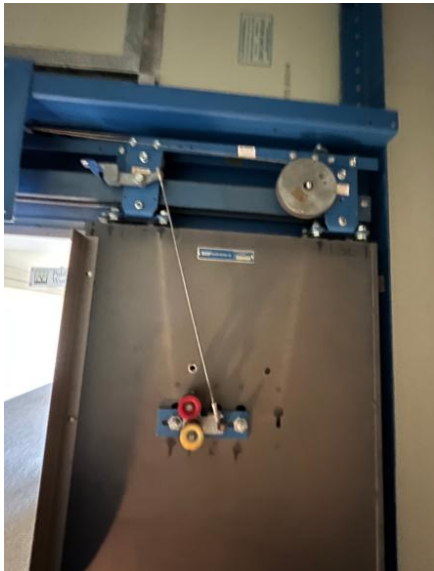
25. City Hall – Car 2 – View from top of the elevator looking at the back of the hall doors. Dover pick up rollers and lock assembly.
