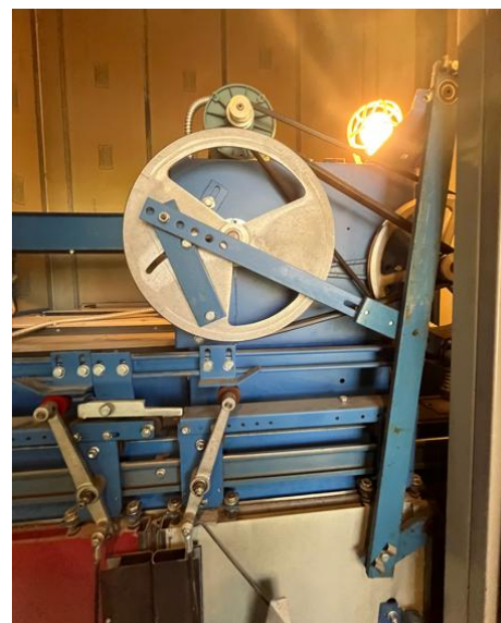
12. City Hall – Car 1 – Dover HD 73 Door Operator.
