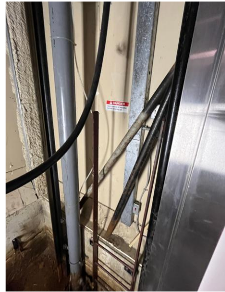
38. Menske Library – View of right side of the pit, hydraulic jack, and pit ladder.
