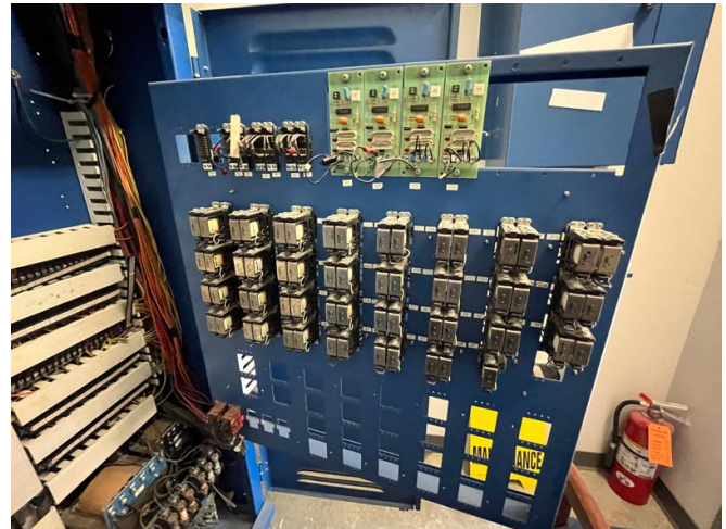
18. City Hall – Car 2 – Inside of WCR controller.
