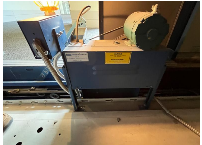
24. City Hall – Car 2 - HD 73 Dover door operator.
