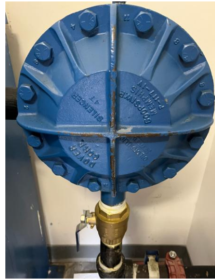
22. City Hall – car 2 – Hydraulic silencer and shut off valve.
