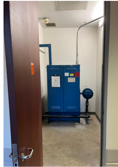
2. City Hall – Car 1 – Machine room and Dover DMC controller.
