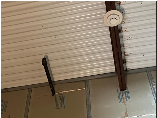
23. City Hall – Car 2 – Top of hoistway. Sprinkler has been capped and smoke in overhead.
