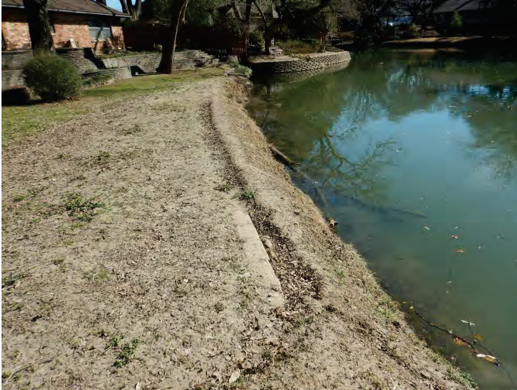
Photo 45. Sediment accumulation along the right bank (photo taken looking upstream along the right bank).
