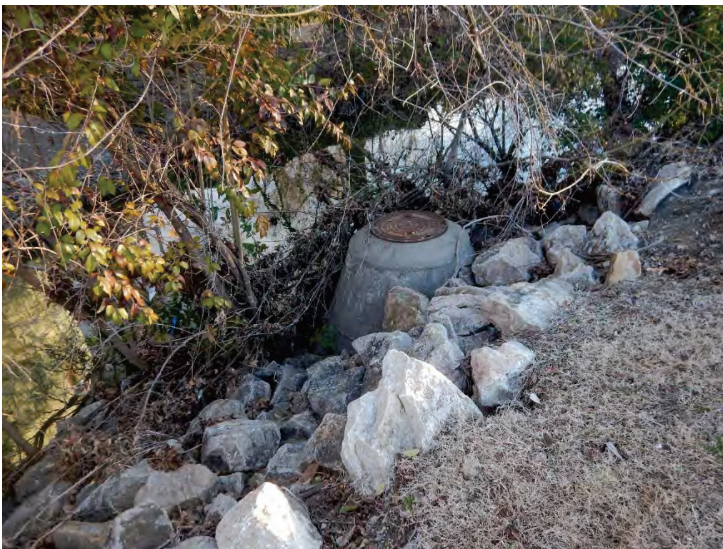
Photo 16. A manhole next to the creek protected with riprap (photo taken looking into the channel from the top of the right bank). This is no immediate threat, but it should be monitored.
