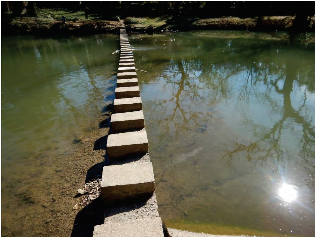
Photo 46. This structure is no longer straight; according to a homeowner, water flows under the dam (photo taken looking towards the left bank).
