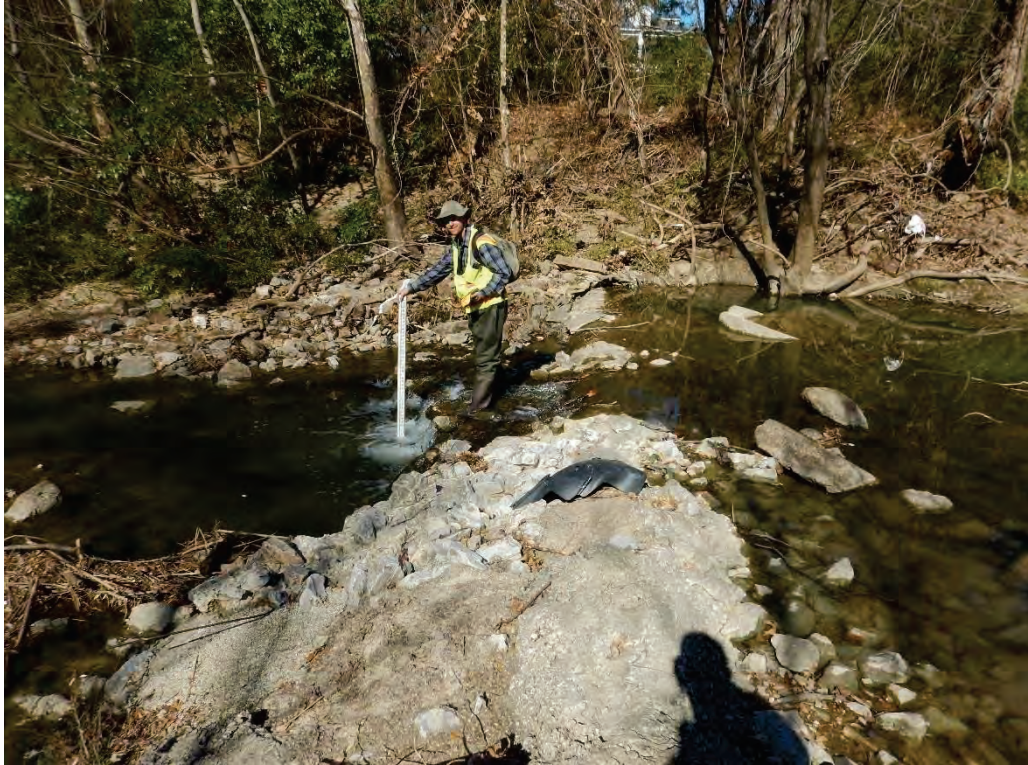
Photo 49. An exposed sewer line with a 2-foot scour hole on the downstream side (photo taken looking towards the right bank).
