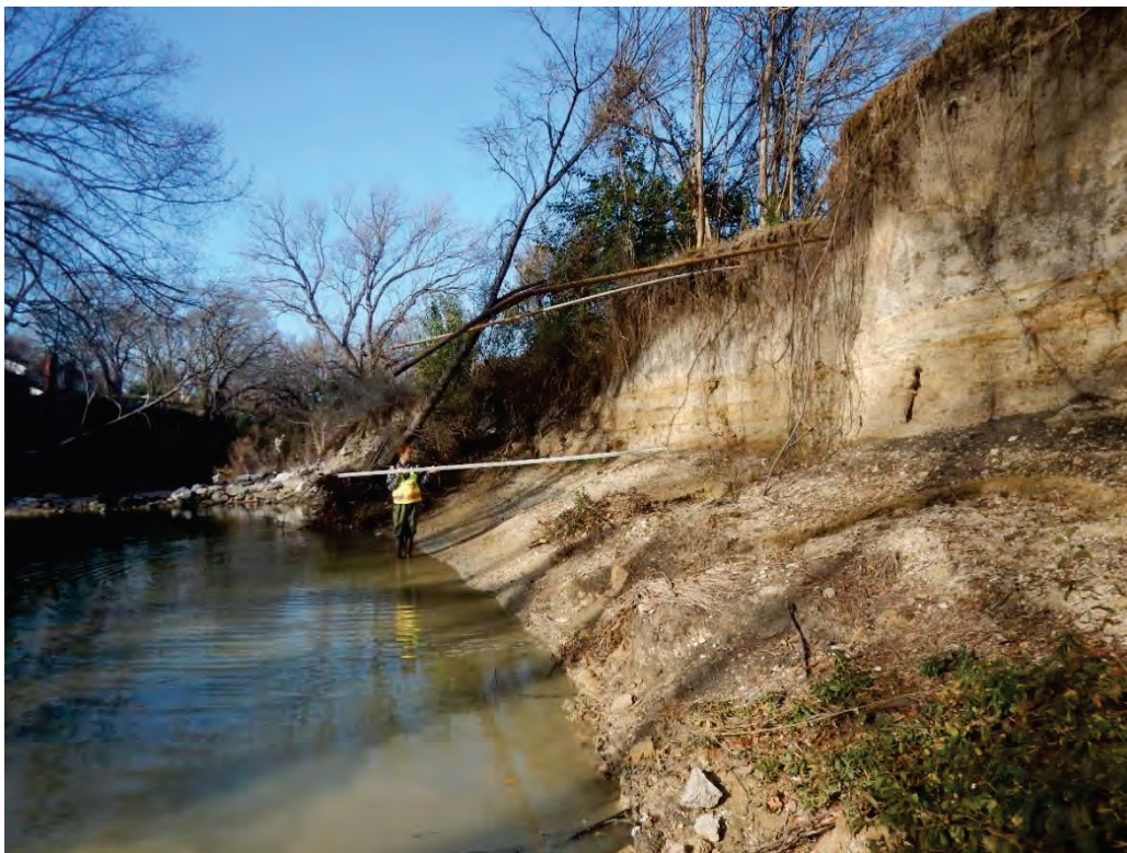
Photo 26. Exposed metal pipes are hanging over 12 feet out of a highly eroded right bank (15 feet tall), indicating the extent of erosion (photo taken looking downstream along the right bank).
