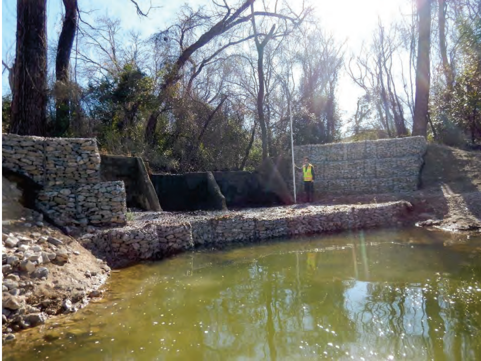
Photo 5. Gabions surround an outfall structure. Erosion of fill could lead to damaged gabions. Consider maintenance to remove excess fill (photo taken looking at the left bank).
