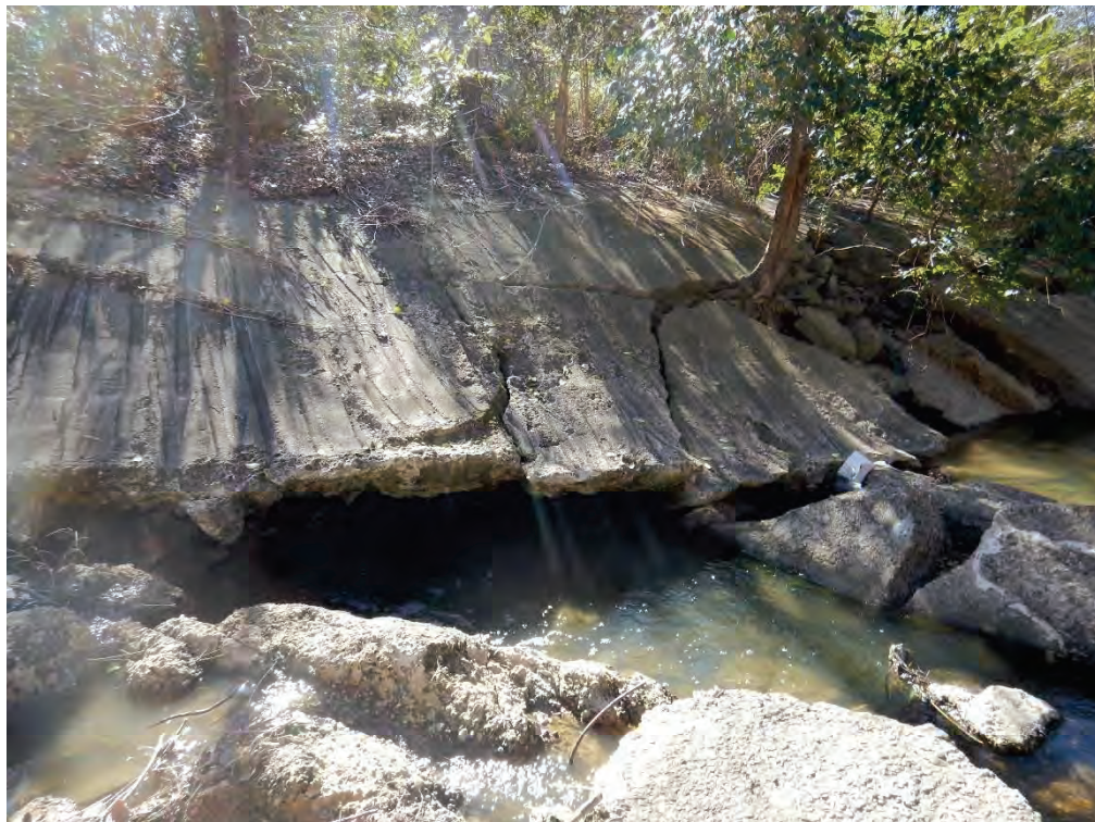
Photo 14. Undercutting (2 feet) of the broken concrete channel lining (photo taken looking at the left bank just downstream of photo 8).
