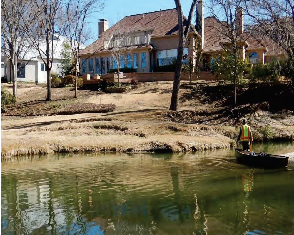
Photo 11. Downstream of the large dam, there is slumping on the left bank. No undercutting was observed (photo taken looking at the left bank).
