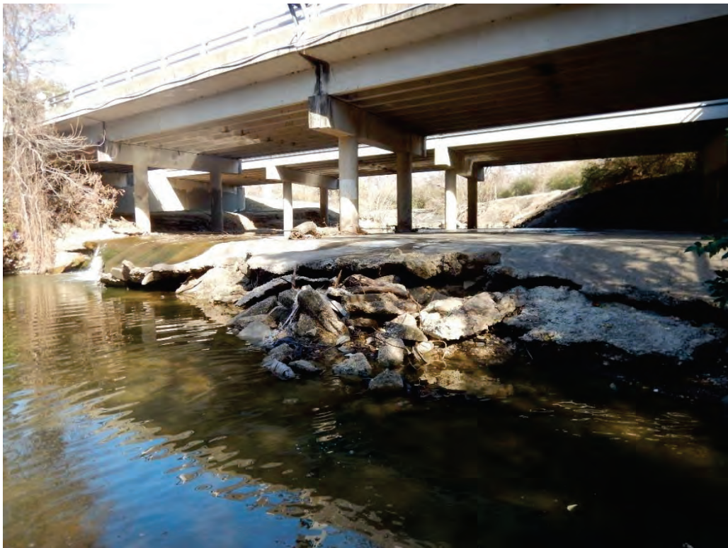
Photo 50. An undercut concrete apron downstream of Ford Road (photo taken looking upstream at the Ford Road bridge crossing).
