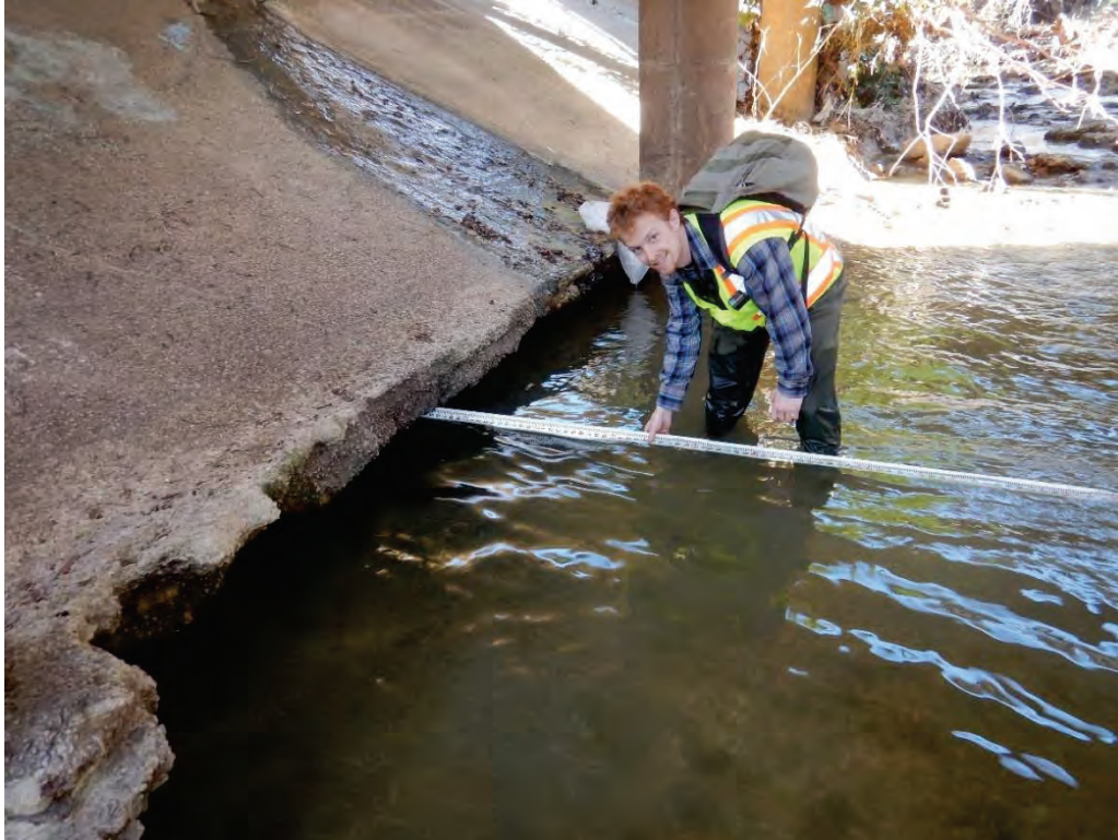
Photo 33. Severe (5.5ft) undercutting of the right bank concrete apron under Webb Chapel Road due to scour (photo taken looking upstream along the right bank).
