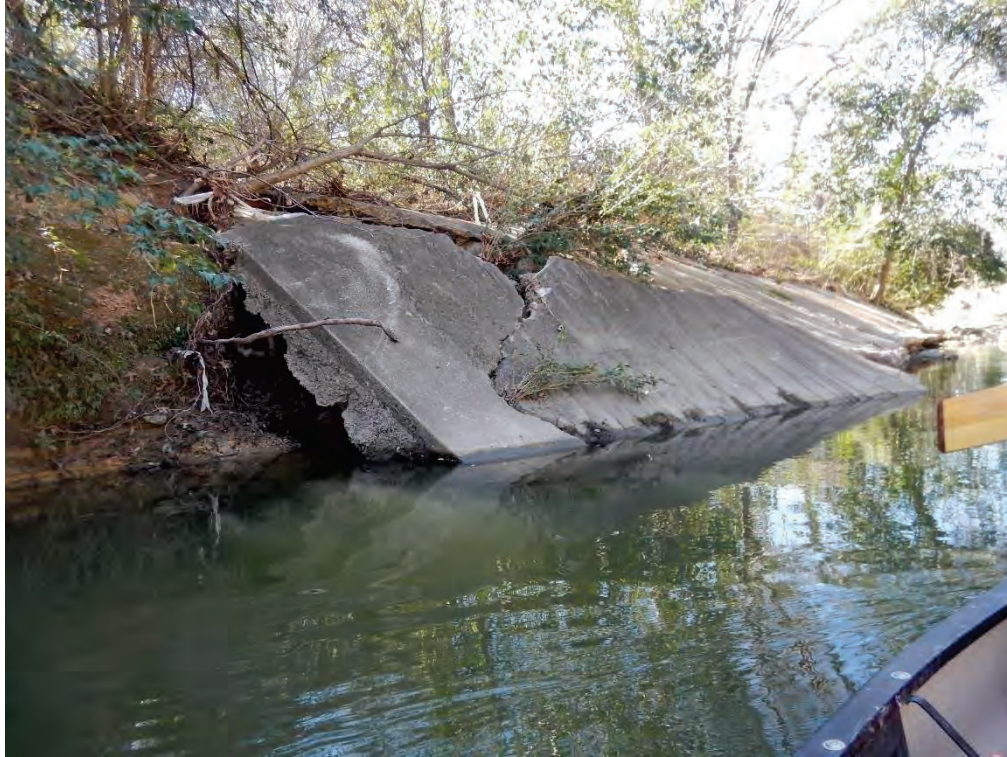
Photo 13. This broken concrete channel lining acts as a grade control (photo taken looking at the left bank).
