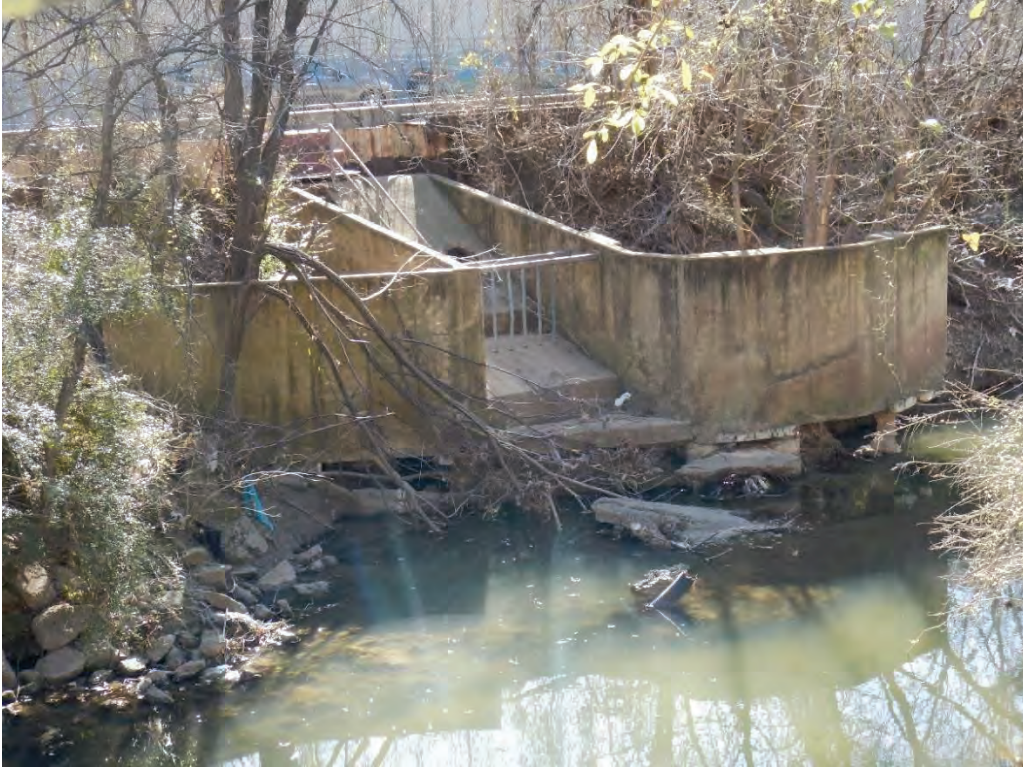
Photo 51. Undercut outfall wingwalls (by 2-3 feet) on the left bank due to scour (photo taken looking at the left bank). It is recommended that an engineer evaluate the condition of this structure.
