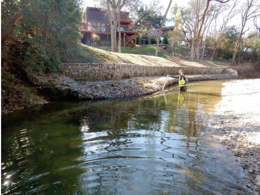
Photo 29. A low gabion basket wall with a mattress toe on the left bank has been undercut ~2ft; the mattress toe is sagging and is missing some rock (photo taken looking downstream along the left bank).
