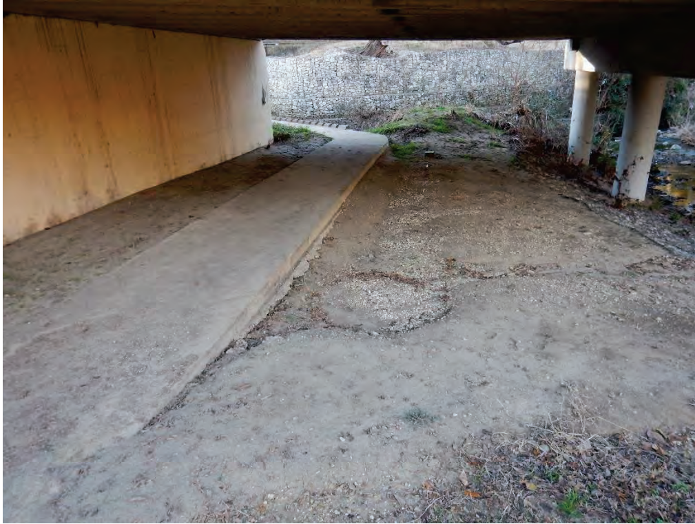
Photo 17. Minor erosion of sidewalk under Valley View Lane (photo taken looking downstream along the left bank). This should be monitored.
