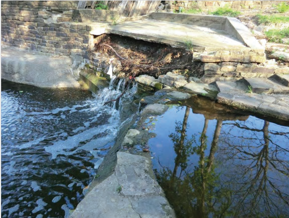
Photo 37. Throughflow behind this training wall is causing erosion and undermining of the structure (photo taken looking at the right bank).
