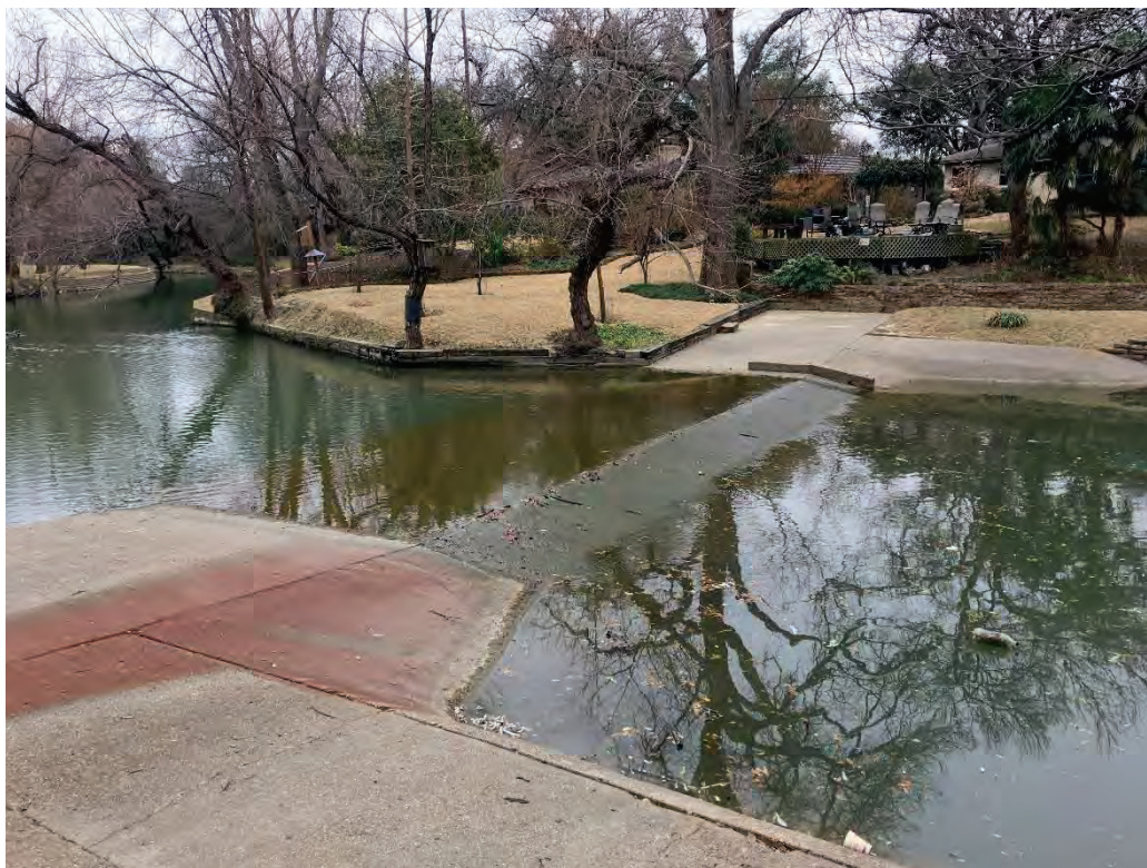
Photo 44. This dam is undercut 2-3 feet. At high flows, water flows quickly over this structure and into the far bank, causing erosion (photo taken looking at the left bank).
