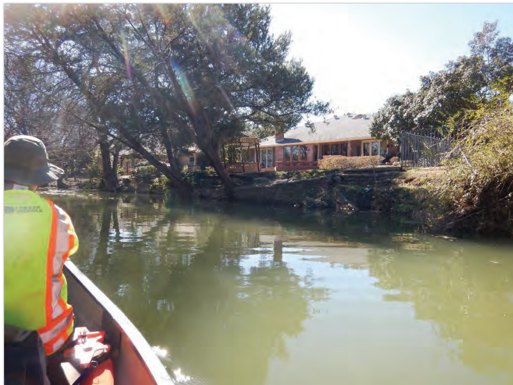
Photo 10. A bag wall on the right bank is collapsing; trees are leaning over the creek. Monitoring or maintenance is recommended (photo taken looking at the right bank).
