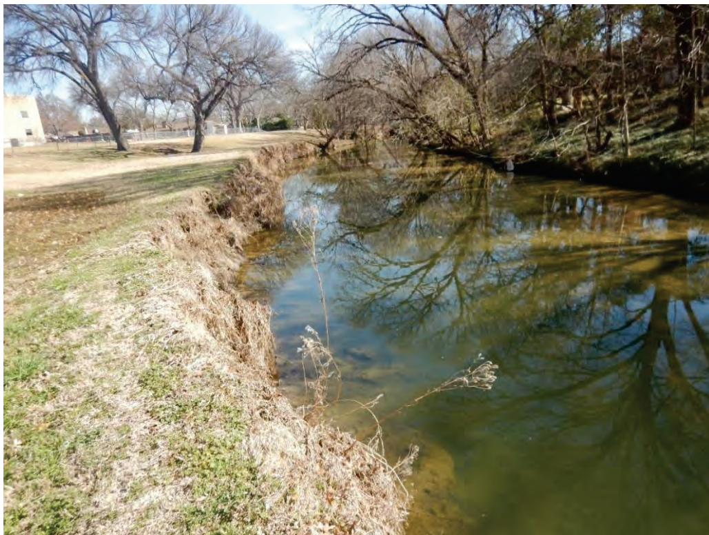
Photo 42. High erosion at Stark Elementary (photo taken looking upstream). The grass is mowed to the top of the banks.
