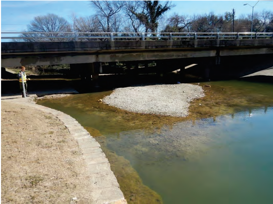
Photo 43. Sediment deposition extends into the pond at Mallon Park (photo taken looking upstream at Josey Lane [upstream end of the pond]).
