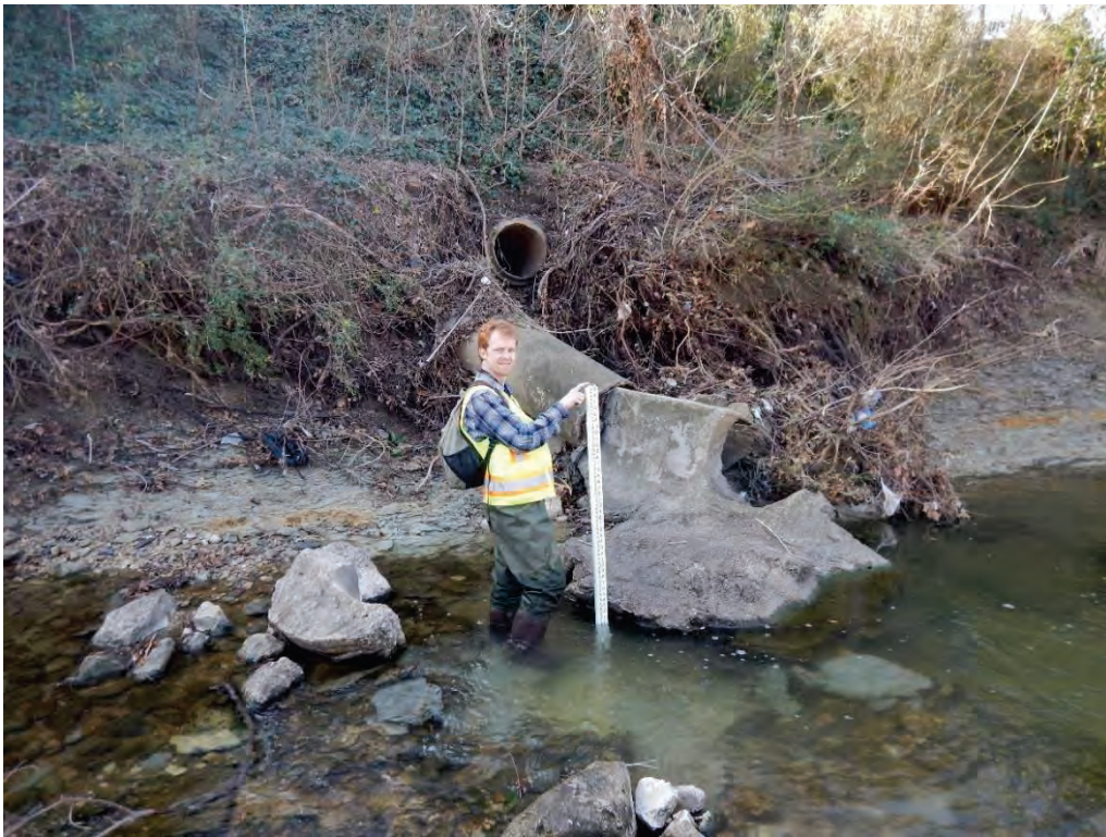
Photo 28. A headwall and outfall pipe on the left bank have collapsed due to channel widening (photo taken looking at the left bank).
