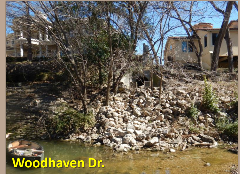
Rip Rap Outfall Protection
