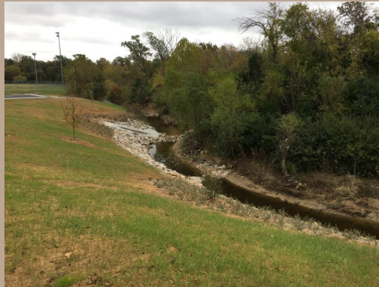
Stabilized Vegetated Bank with Rock Toe
