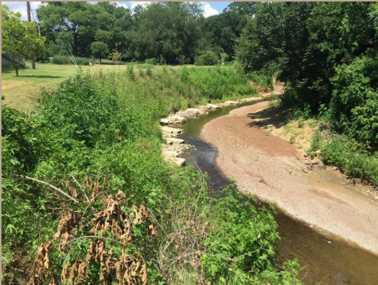
Stabilized Vegetated Bank
