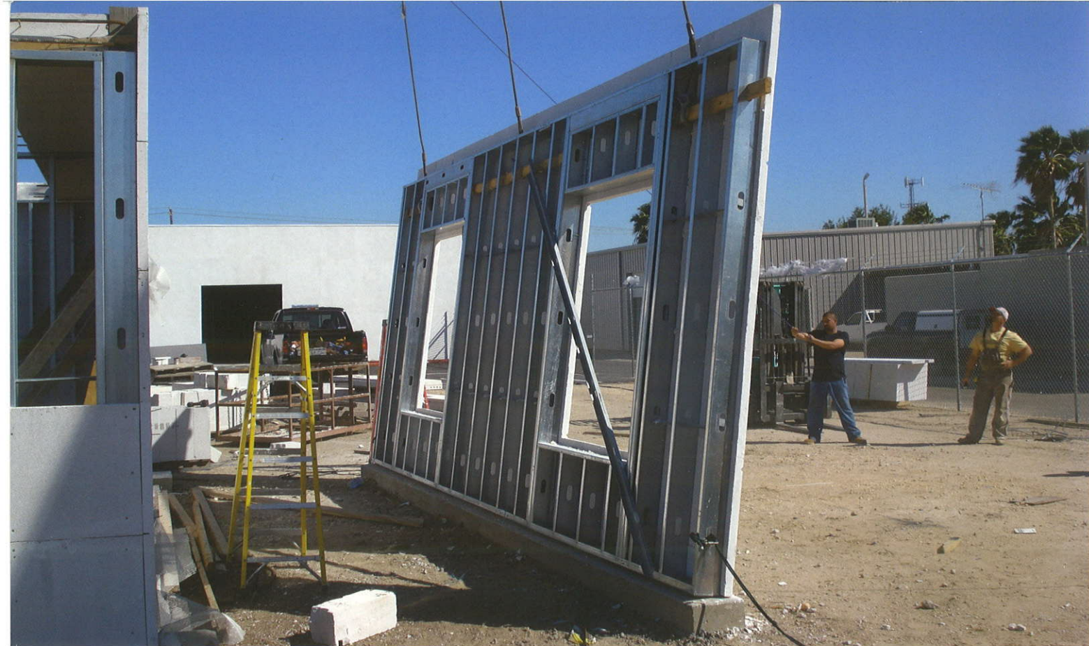
Prefabricated metal stud walls sheathed with two inch Hebel Autoclaved Aerated Concrete (AAC) Panels, plastered and painted. Erected as an architecturally finished curtain wall. Hebel Metal can be finished very easy with any type of finish systems meeting any architectural requirements.
