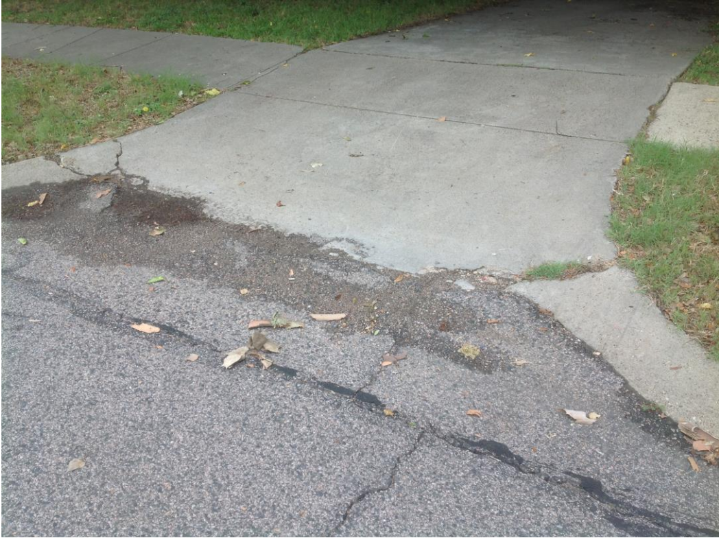
Spalling driveways
