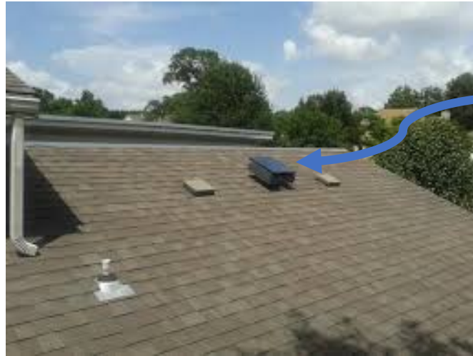
Picture of Solar Vent Fan installed on a roof
