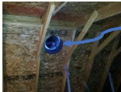
Picture of inside of roof of installed Solar Vent Fan
