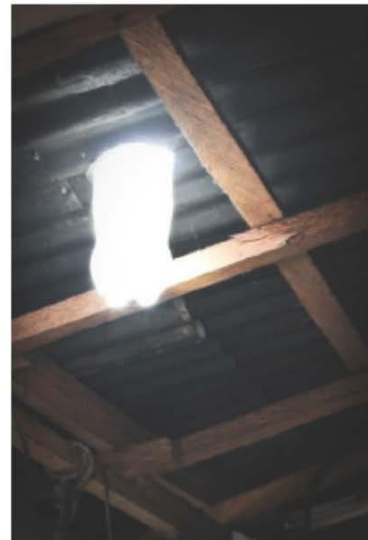
Inside of shed with Solar Bottle Bulb
