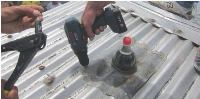
Solar Bottle Bulb – Exterior Roof
