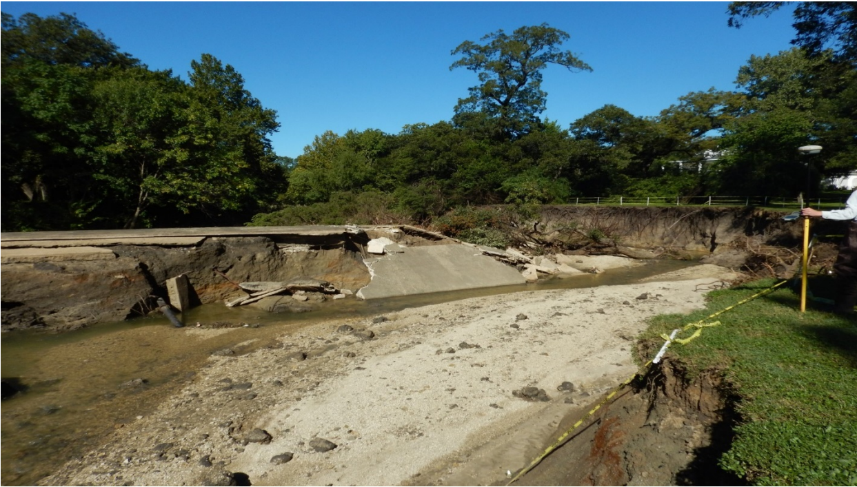
Failed Bonneau Dam – Before Emergency Work
