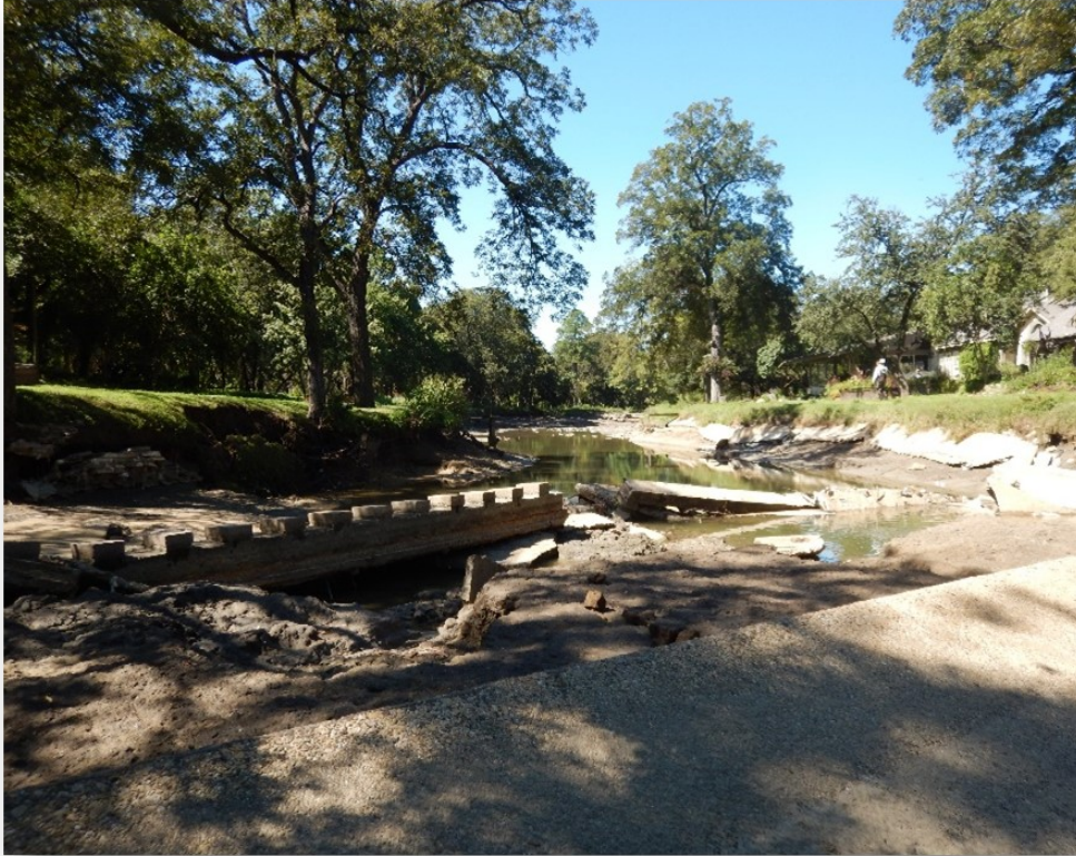
Failed Secondary Dam – Before Emergency Work
