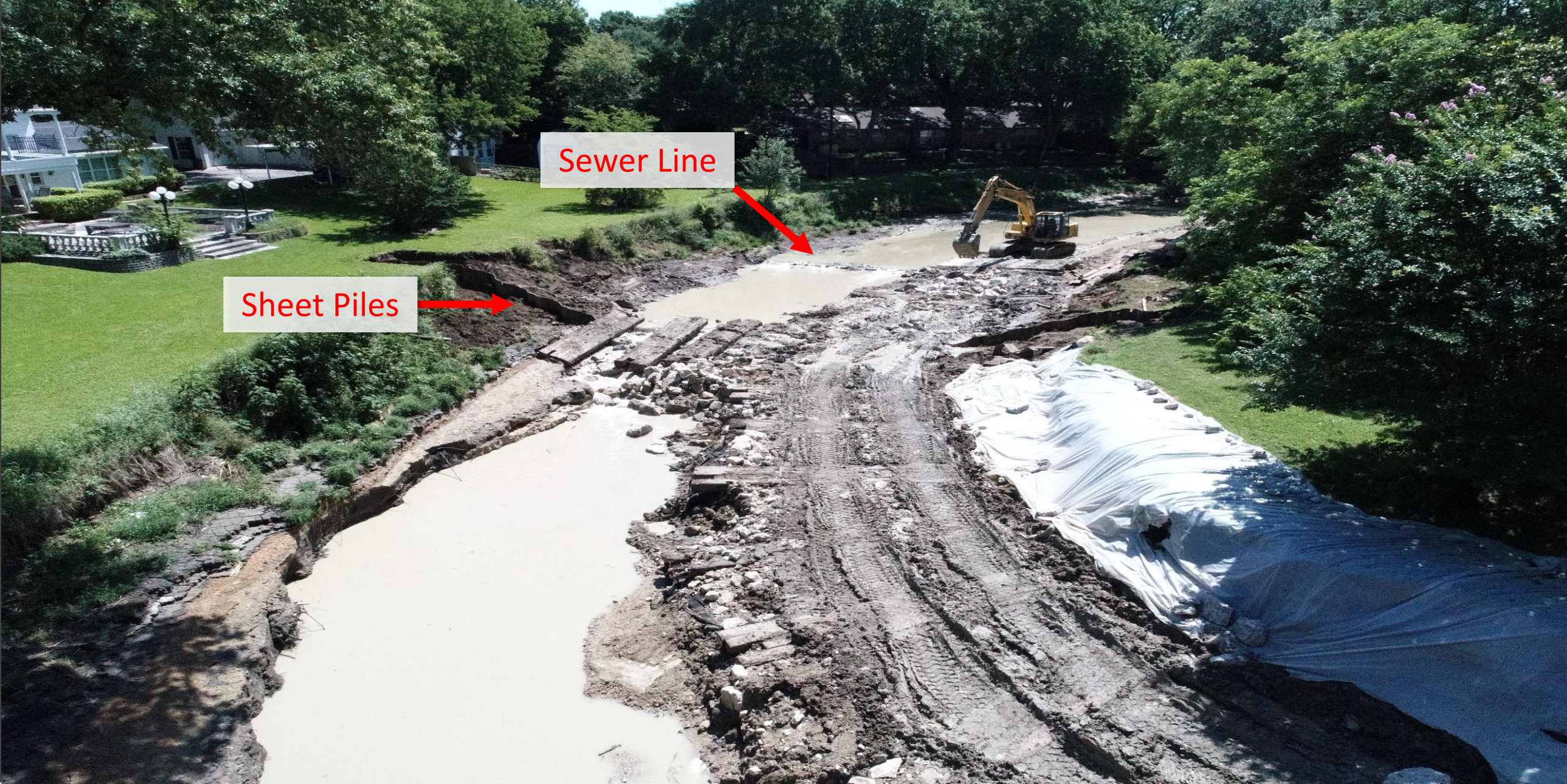
Sheet Pile Drop Structure Under Construction
